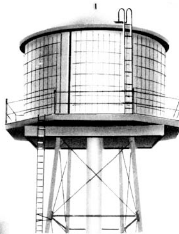
WOOD TANK ON TOWER
