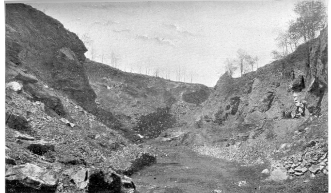
OPEN PIT, JACKSON IRON MINE.
