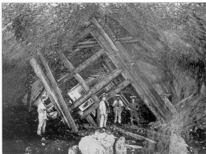
SHOWING TIMBERING IN CALUMET & HECLA COPPER MINE.
