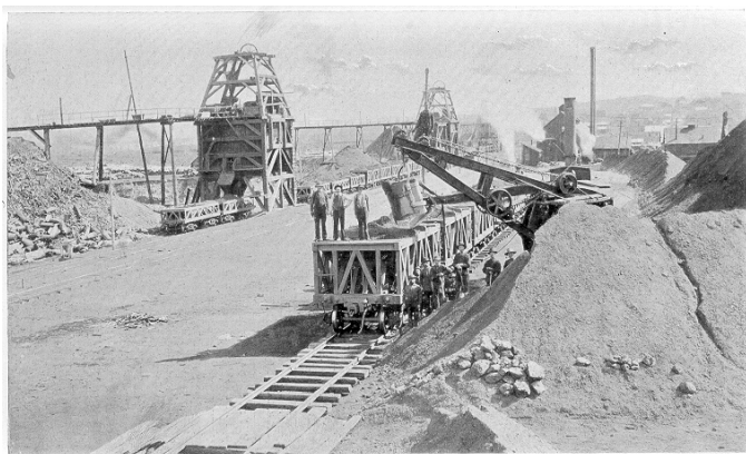
SHAFTS AT EAST NORRIE MINE.
