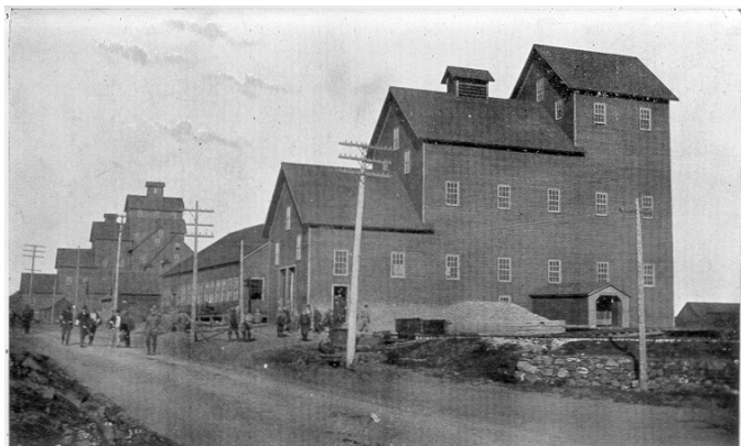
SHAFT AND ROCK HOUSES, QUINCY MINE, HANCOCK.
