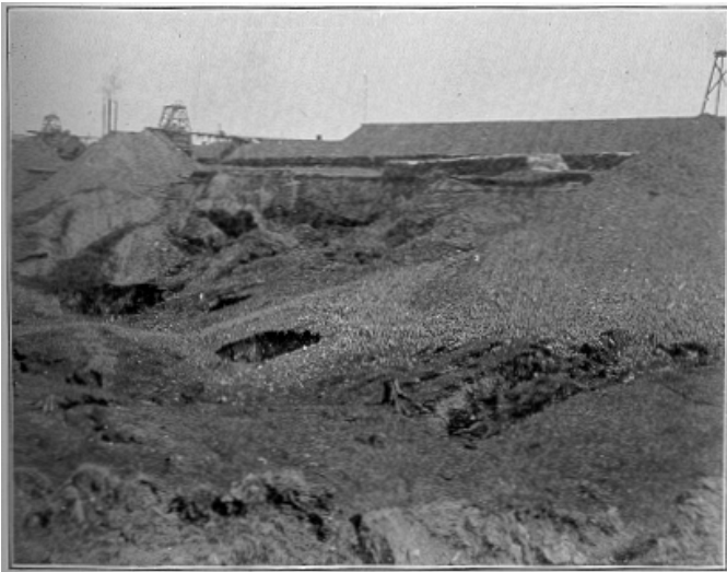
SHOWING CAVING GROUND, NORRIE MINE.
