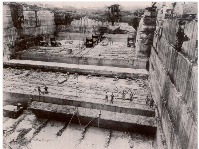
Figure 1. - Blocks of dimension limestone turned down ready for subdivision.
