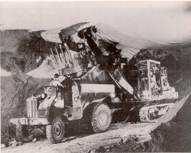
Figure 3. - Electric shovel with 1-½-yard bucket, loading limestone into a diesel-powered truck in Barberton, Ohio.
