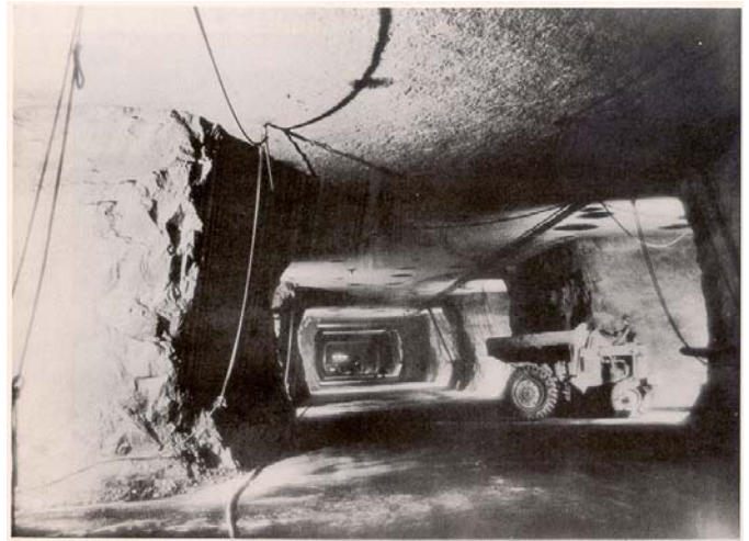
Figure 4. - One of the diesel-powered trucks used for hauling limestone from working faces to shaft in Barberton, Ohio.
