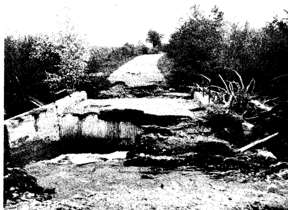
Culverts, bridges, and roadfill yielded to the raging waters.
