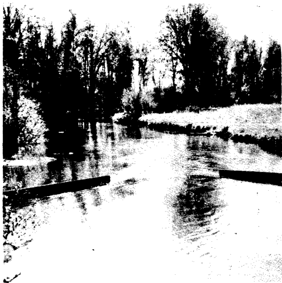
FIGURE 62.--Jetties deflect eroding currents and arrest the decay of stream banks.
