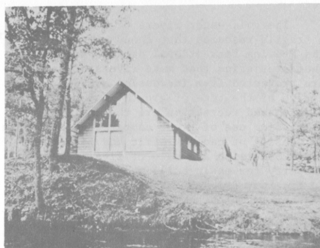
Grading the lot at this cabin allows silt and sand to wash into the river.
