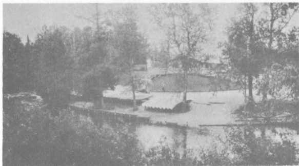
Canoe Livery landing on Manistee River. Bank is protected by wood sheet piling for boat dockage.
