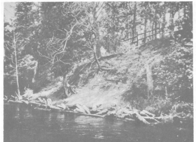
Figure 68. Rip rap of logs and stumps protects the base of a high sandy bank at this campsite on the Au Sable below Grayling. Upper slope is eroding because some campers still climb up and down banks to enter and leave the river.
