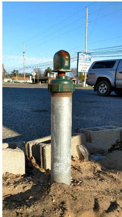
Drilled Well with Steel Casing
