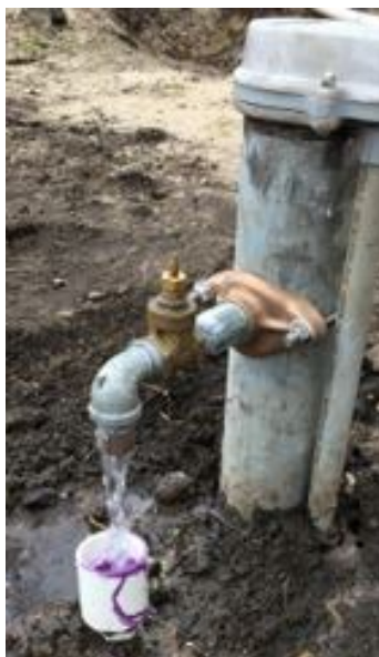
Air Gap on Flowing Well
