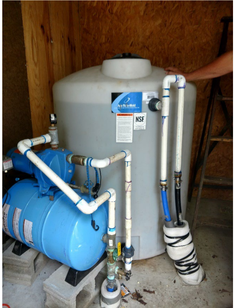
Storage Tank Re-Pump System
