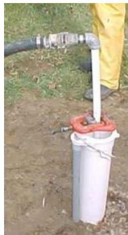
Pumping Chlorinated Water to Bottom of Well
