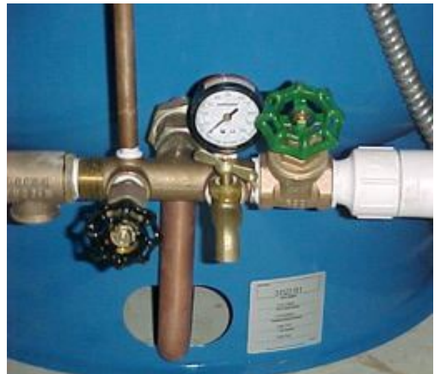
Pressure Relief Valve, Hose Bibb, and Threadless Sample Tap
