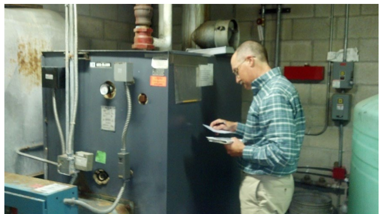
Evaluate Backflow Prevention
