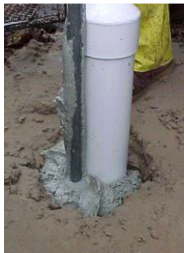
Bentonite Return at Surface
