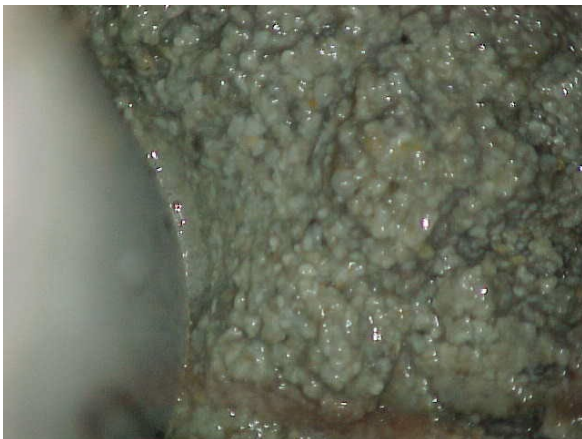
Bentonite Pumped into Annulus
