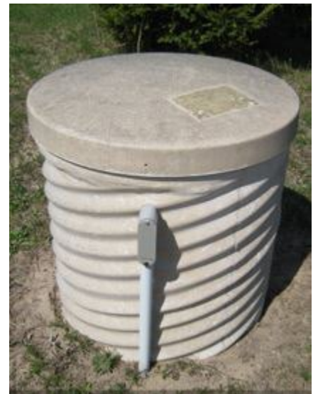
Augered Well with Fiberglass Casing
