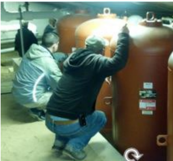
Inspect Pressure Tanks
