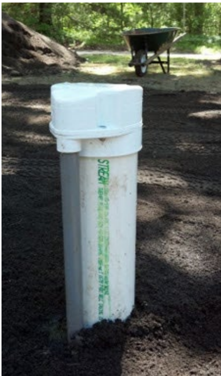
Drilled Well with PVC Casing
