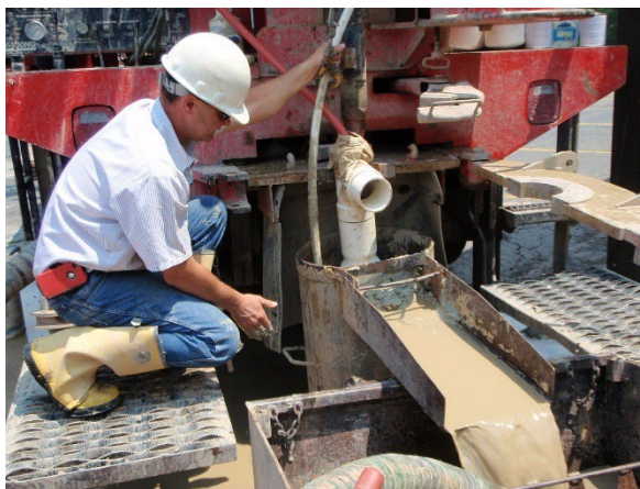
Grouting Annular Space
