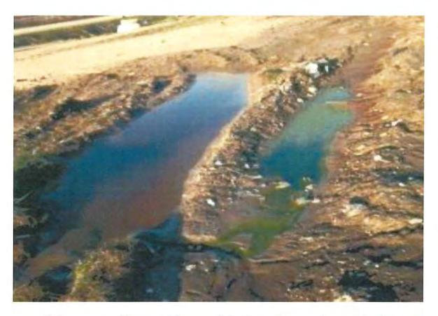
• Daily cover was either not put down on all the three active waste faces or when it was placed, it was not stripped/removed the following morning. It should be noted that Advanced's MDEQ Operations plan specifies at least 6 inches of daily cover placed each day. Failure to strip daily cover contributes to watering in wells because leachate is prevented from draining down the waste mass as intended where the Landfill is designed to collect.
