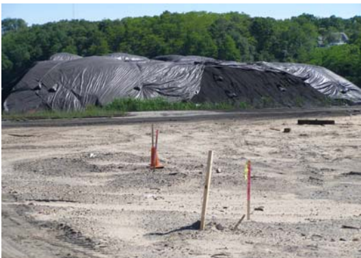
Aggregate Storage Area (Before)
