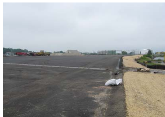
Aggregate Storage Area (After)
