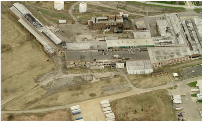
Building 2 was used for papermaking, dyeing, coating, and cutting. (Before)
