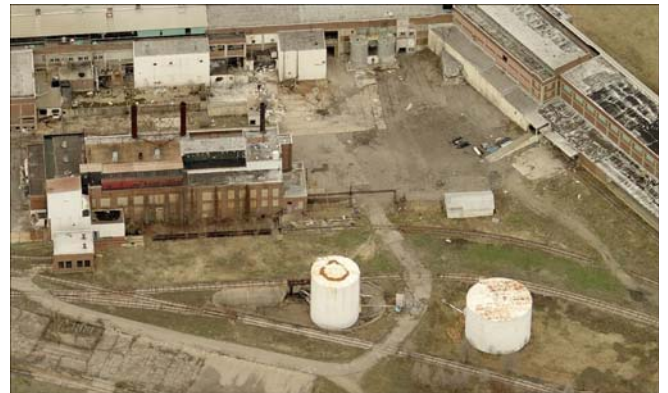
The mill's power plant (Before)
