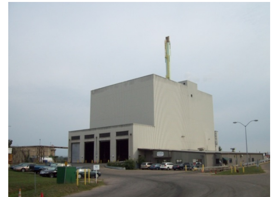
Above: Municipal solid waste incinerator
