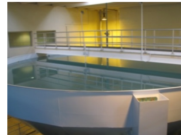
Left - WWTP Clarification Tank
