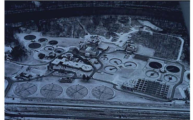
Above - Aerial of a Waste Water Treatment Plant (WWTP)
