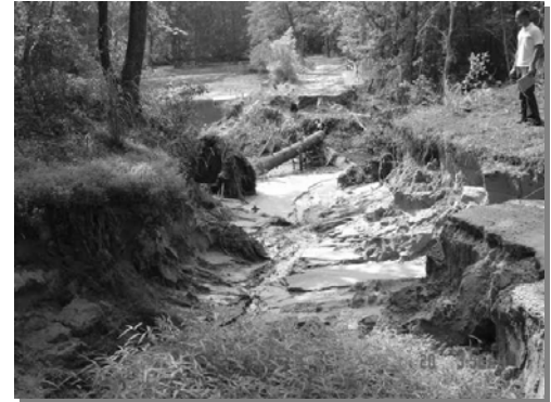
Erosion from Uprooting of trees
