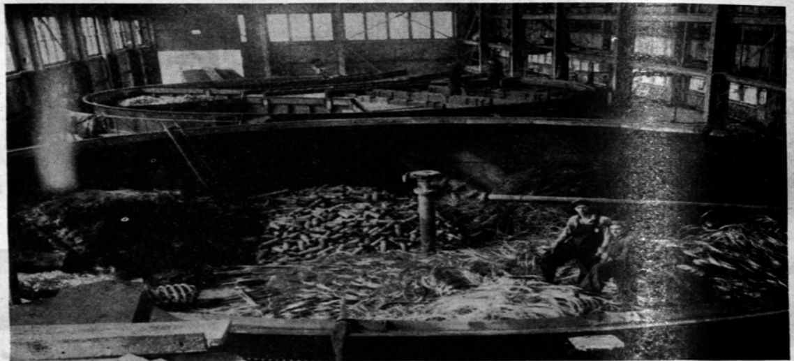
LOADING SECONDARY COPPER into tank for leaching at Tamarack reclamation plant at the Calumet & Hecla Consolidated Copper Co. plant. Subdivided tank in the background is used to treat lots separately. See article on operations p. 89.
