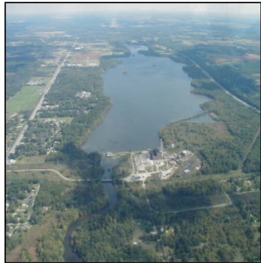
Figure 1-2. Morrow Lake Upstream of the API/KR/PC Superfund Site.
