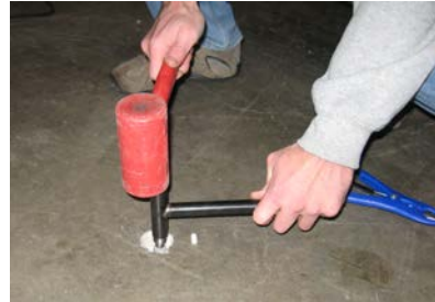
Figure 5. Tap Vapor Pin™ into place.
