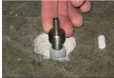
Figure 4. Place Vapor Pin™ in hole.
