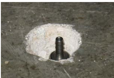
Figure 6. Installed Vapor Pin™.
