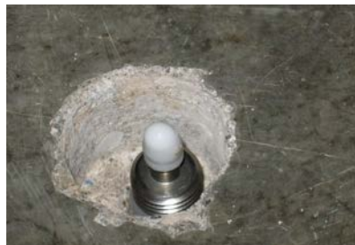
Figure 7. Place Protective Cap.
