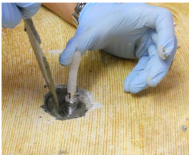
Figure 6. Seal annular space
