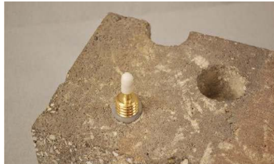
Figure 9. Temporary Vapor Pin™ Installation.
