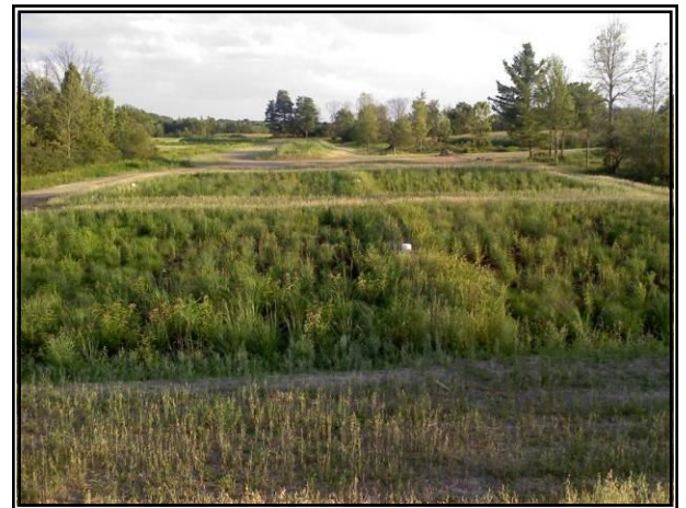
Site Conditions After Construction: View of constructed lined wetland cells with established vegetation.
