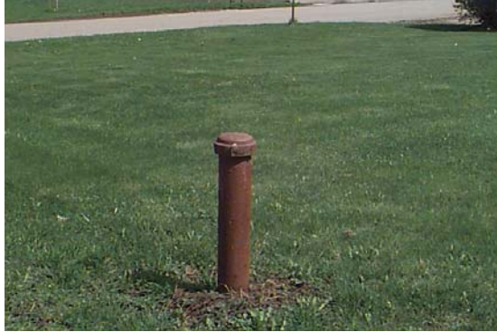
Typical wellhead for small diameter well.
