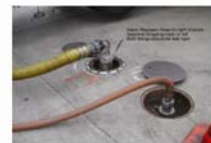
FIGURE 8. Dropping a load of gasoline with a dual-point connection.
