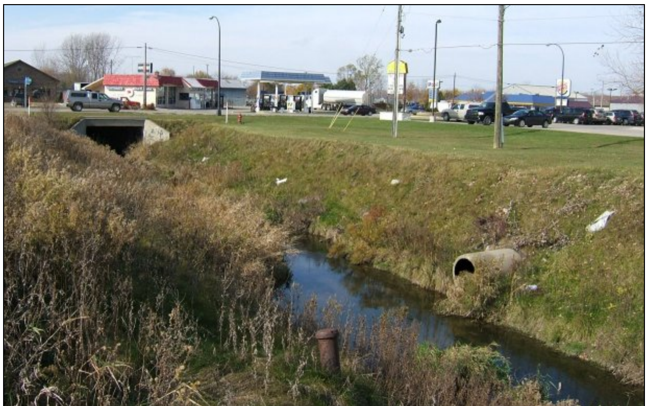
Figure 22: Bad Axe Drain at M-53 (Van Dyke Road)
