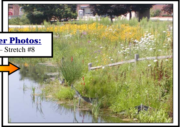
Stabilized stream banks and native riparian buffer vegetation (seed and plugs).
