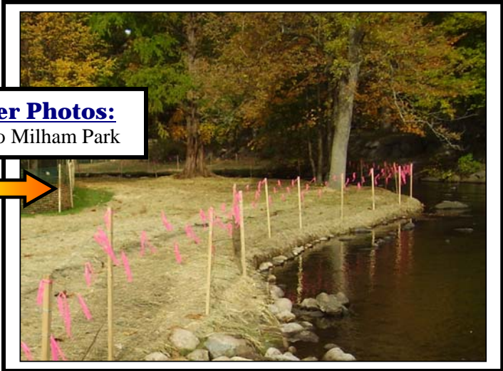
Stabilized stream banks and native riparian buffer vegetation (seed and plugs).
