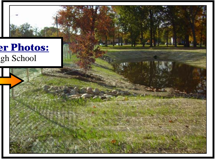
Stabilized stream banks and native riparian buffer vegetation (seed and plugs).
