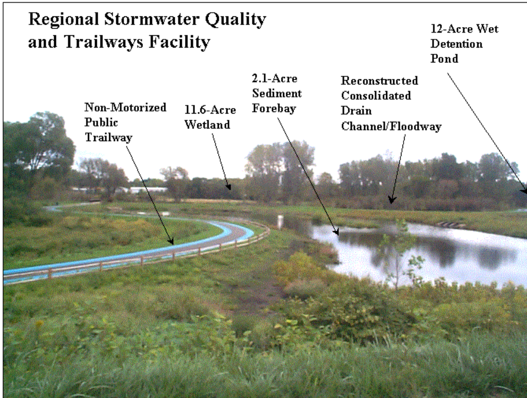
Figure 1. Storm water BMPs installed in Consolidated Drain #1.
