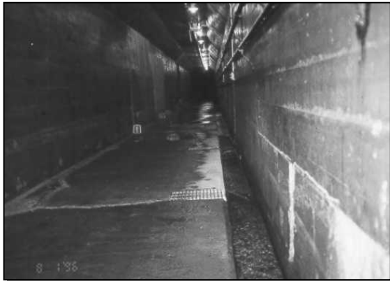
Drainage Galleries/Drain Systems
