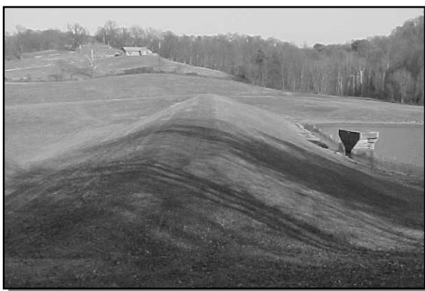
Earthen Embankment Dam
