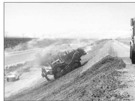
Repair Embankment
