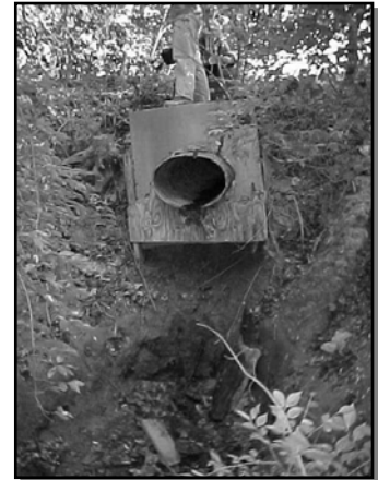
Undermining of Outlet Conduit
