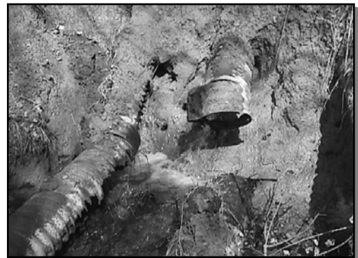
Corrugated Metal Pipe (CMP)
