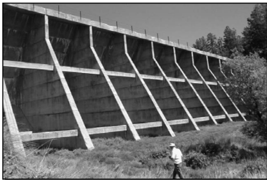
Concrete Buttress Dam
