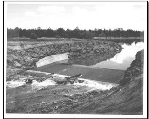
Unlined Earthen Channel Spillway Erosion
