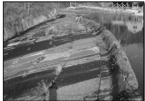
Deterioration of concrete and joints on concrete lined spillway channel
