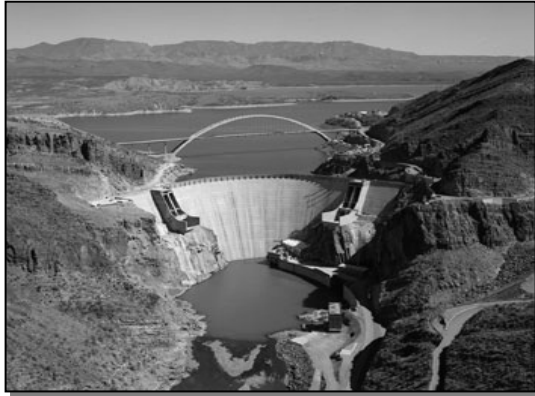
Concrete Arch Dam
