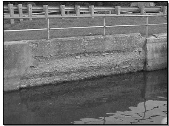
Concrete Spalling
