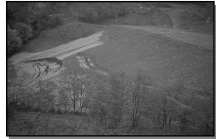
Deep Seated Slope Failure
