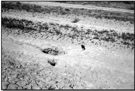
Sinkhole/Dropout
