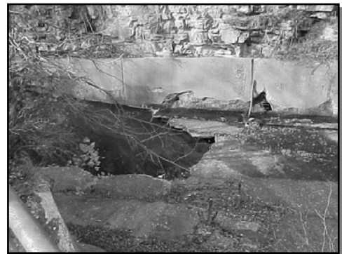
Undermining of concrete slabs on concrete lined spillway channel
