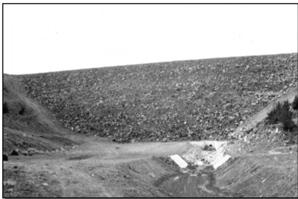
Earth and Rockfill Embankment Dam
