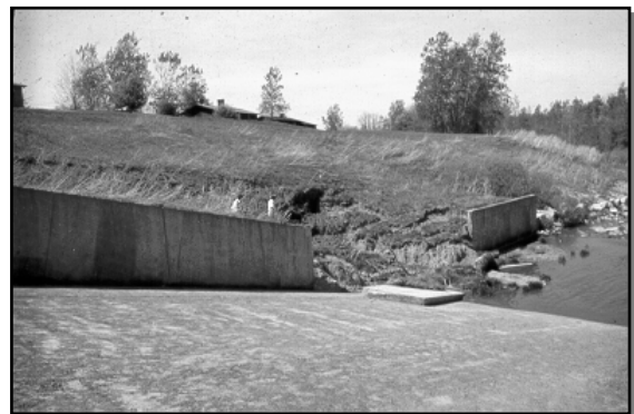
Structural movements - lateral movement
