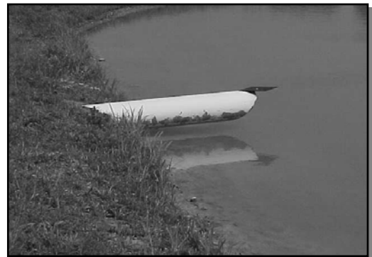
PVC Spillway Pipe
