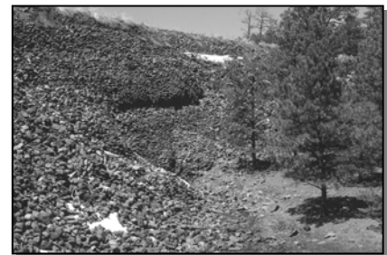
Shallow Slope Failure
