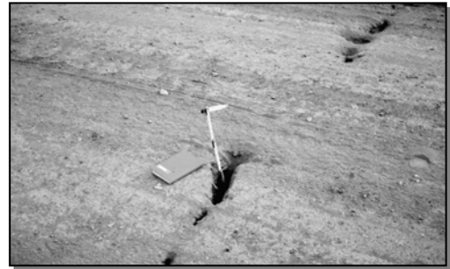
Embankment Cracking
