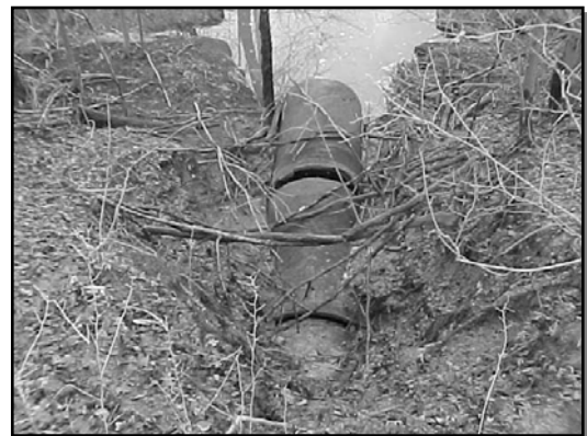
Joint Separation of Outlet Pipe
