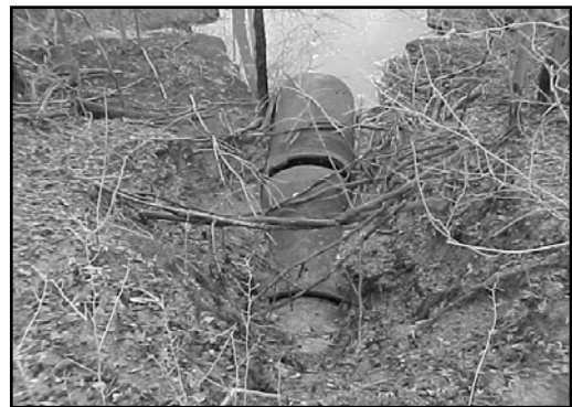
Severe outlet deterioration
