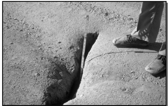
Large crack in the embankment
