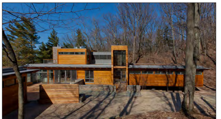
Green roof used to moderate heating and cooling, and extend life of roofing. [8]
