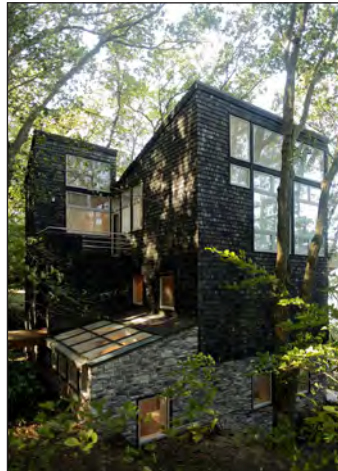
View from North
