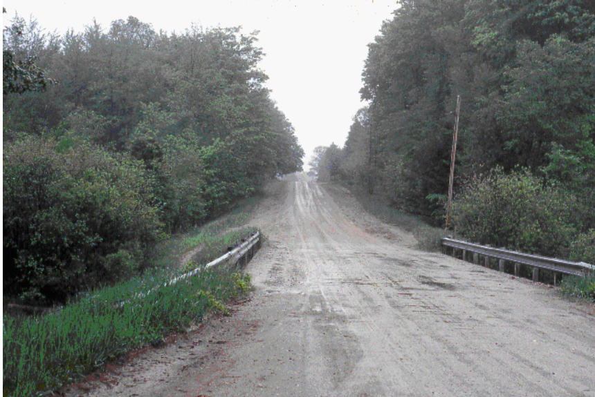
Figure 1. Runoff from steep approaches on dirt roads can cause large amounts of sediment to enter watercourses during rain or snow melt.
