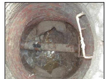
Broken Sanitary Sewer Line Passing through a Storm Drain Discharging to the Middle Rouge River
