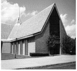
The plank-and-beam method of construction uses beams of significant size to provide a framework which then is covered with thick planks that span the framework. While this method construction is similar to post-and-beam construction, where a rigid frame of posts and beams essentially can stand alone due to the interconnections of the beams and posts, plank and
