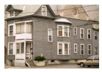
Balloon-frame construction was first used about 1833, and became a very popular method of wood-frame construction until about 1950. The advent of sawmills around 1833 opened the way for long and evenly shaped pieces of lumber which were needed for balloon-frame buildings.
