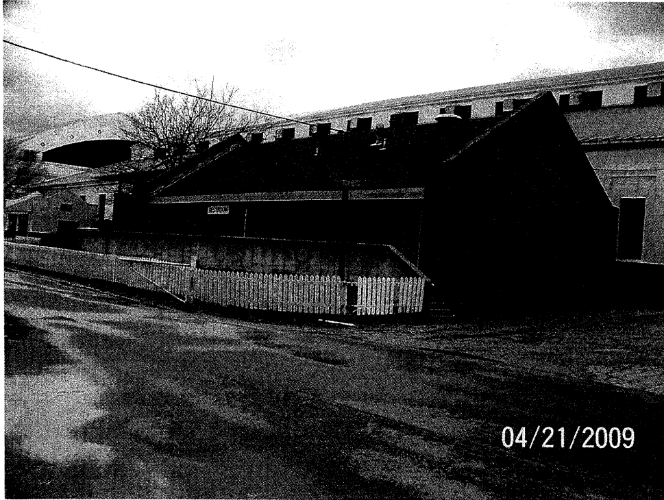
Photograph No. 25: Exterior view of the North Restrooms with the Dairy Cattle Building adjacent and behind.
