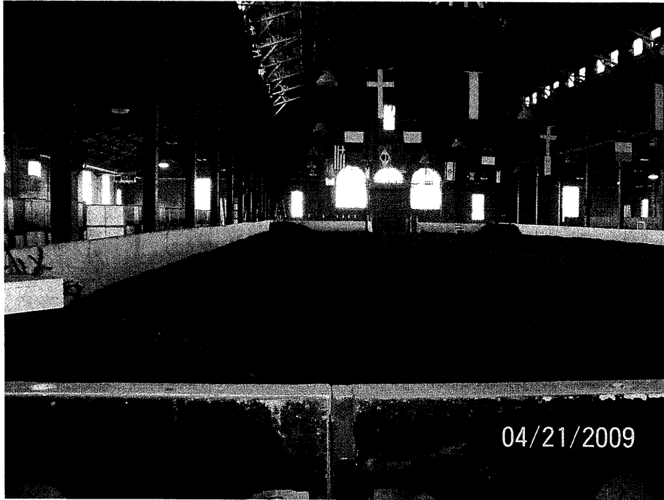
Photograph No. 23: View from south looking north at the riding arena of the Dairy Cattle building.
