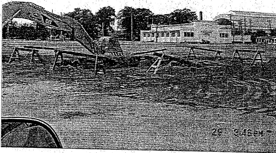
Photograph 20: July 29, 2003 Backfilling of the excavation.
