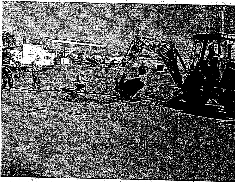
Photograph 2: July 23, 2003 – M.L. Chartier is exposing the UST to pump out tank contents.
