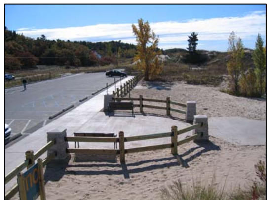
Walkway and parking improvements
