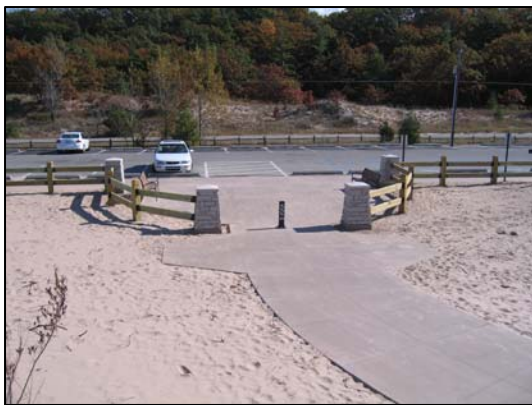
Walkway and parking improvements
