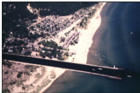
Aerial View of Charles Mears State Park
