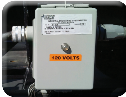
Over night heating system
