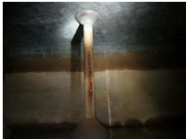
Column Deterioration and Corrosion
