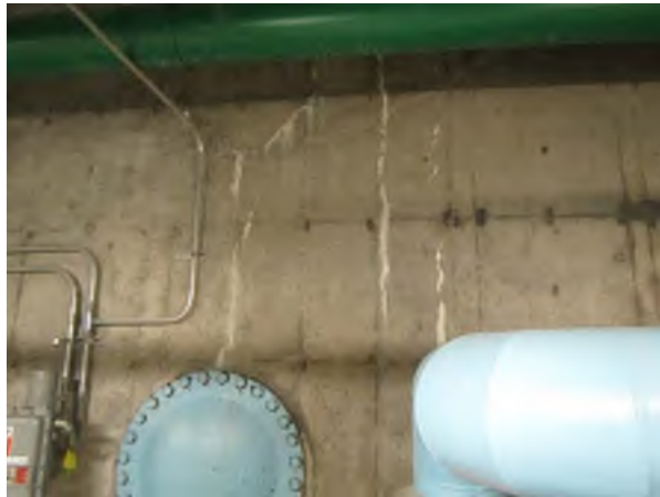
Filter Box Wall Cracking (as seen from Pipe Gallery)
