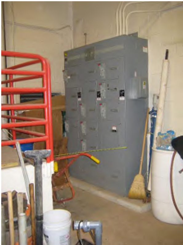
Square D MCC-BB1 that was not Updated with Allen-Bradley in 2014
