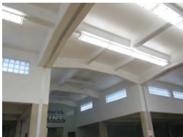
Filter Building, Center Area Roof
