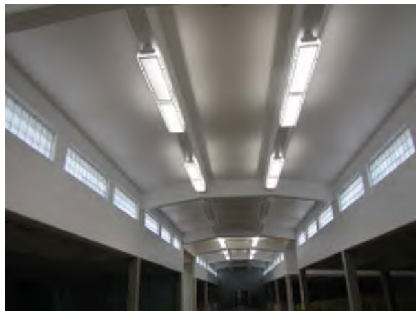
East Filter Gallery Roof Framing, Looking East
