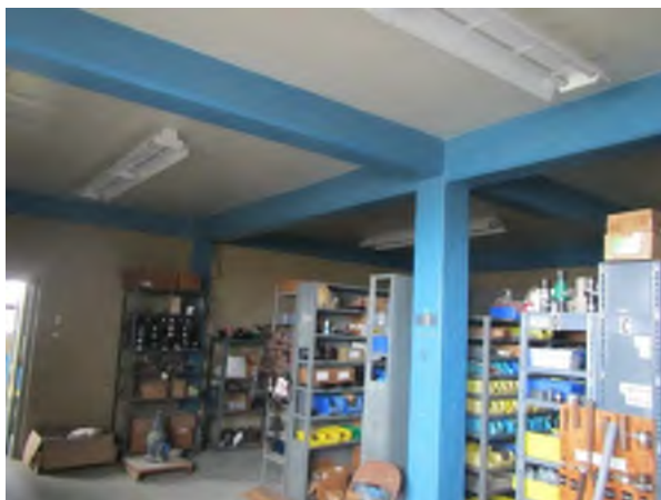
Upper Level Maintenance Storage Room
