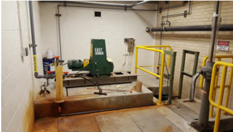
Figure 4.10 – Flint WTP Rapid Mixer Room
