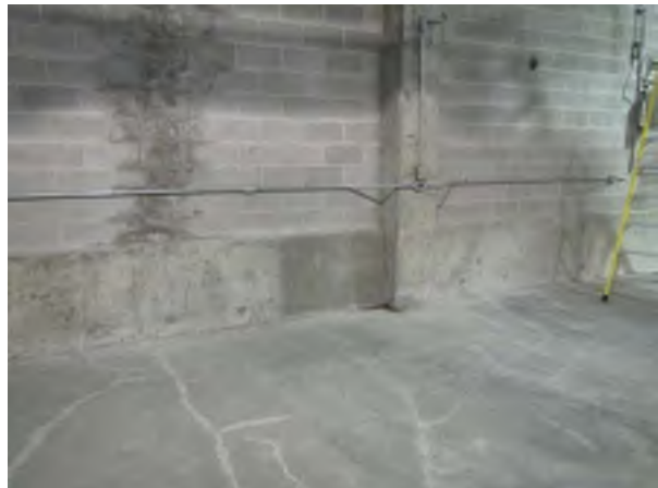
West Exterior Masonry Wall Discoloration, Upper Level
