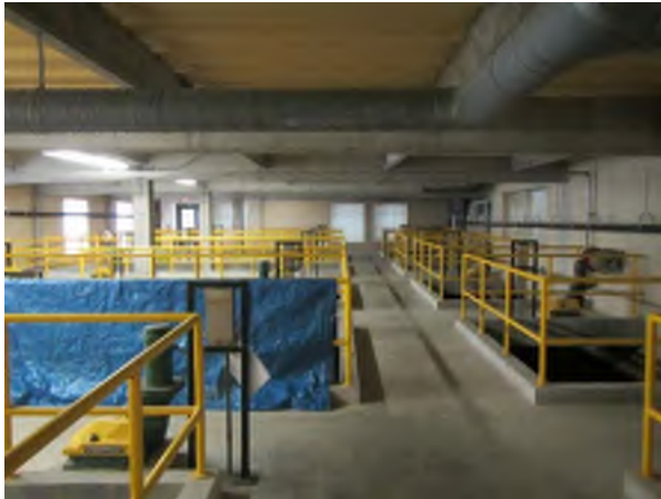
East Flocculation Room
