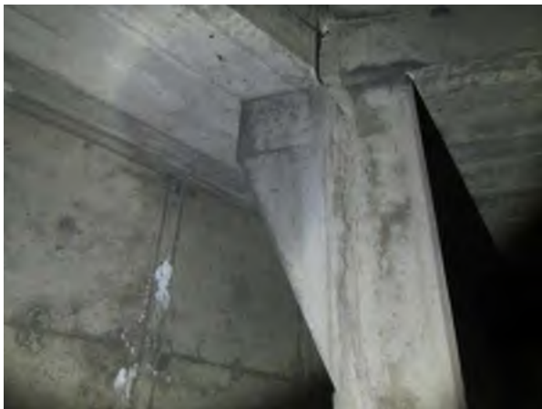
Cracked Column Corbel
