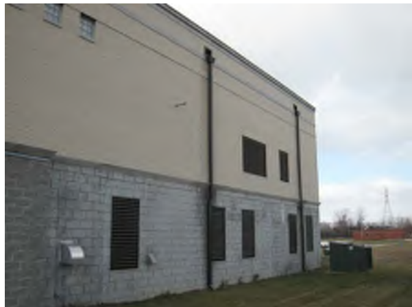
Ozone Building East Wall
