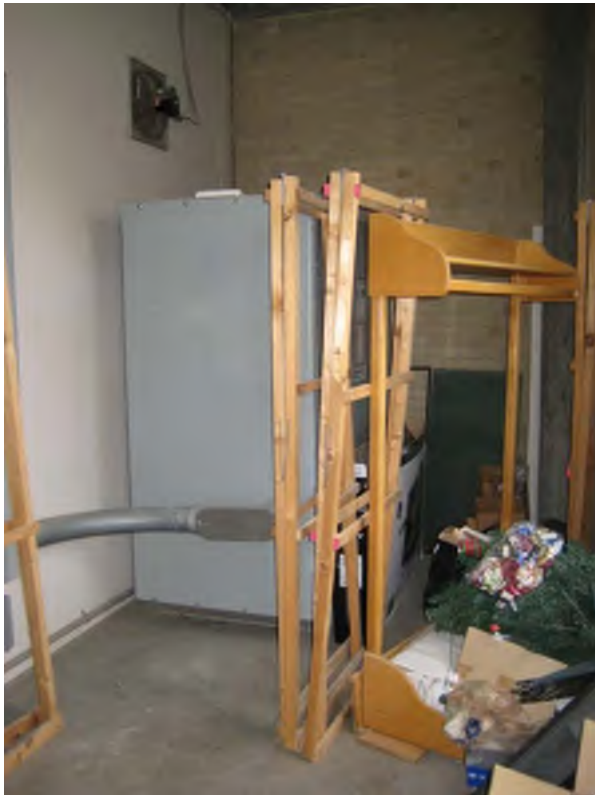
Single Transformer Feeding the Kitchen Electrical Room
