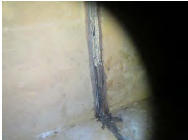
Deteriorated Expansion Joint
