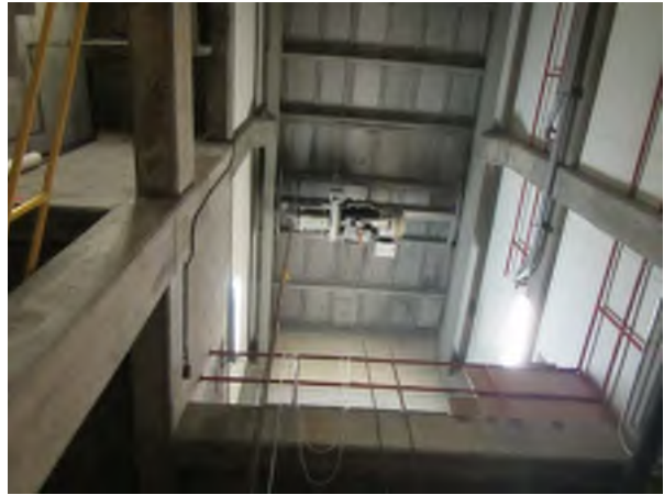
East Loading Area Roof
