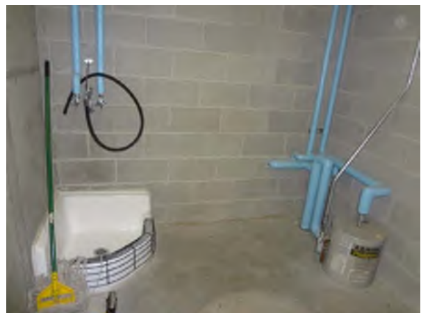
Janitor Room in Ozone Building
