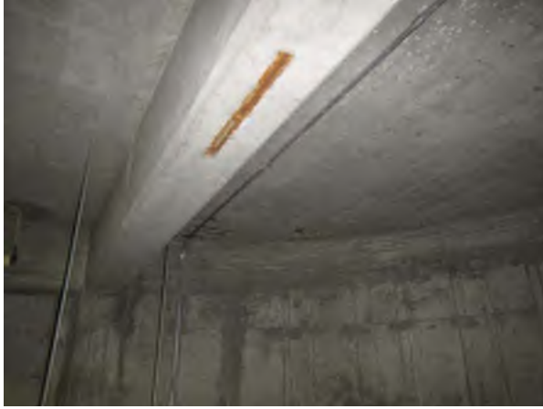
Main Entrance, Underside of Elevated Slab, Corroded Steel Insert Embedded in Beam
