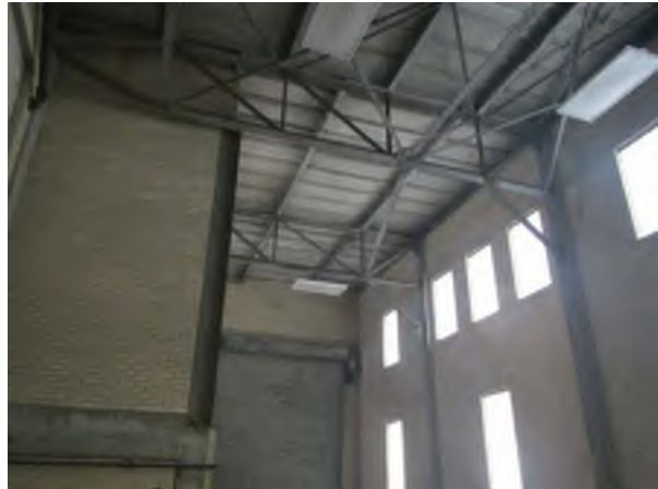
West Loading Building, Looking South
