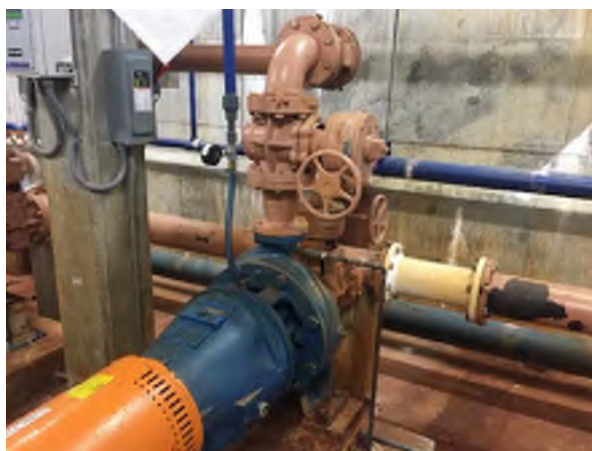
Isolation and Check Valves for Sludge Pumping System
