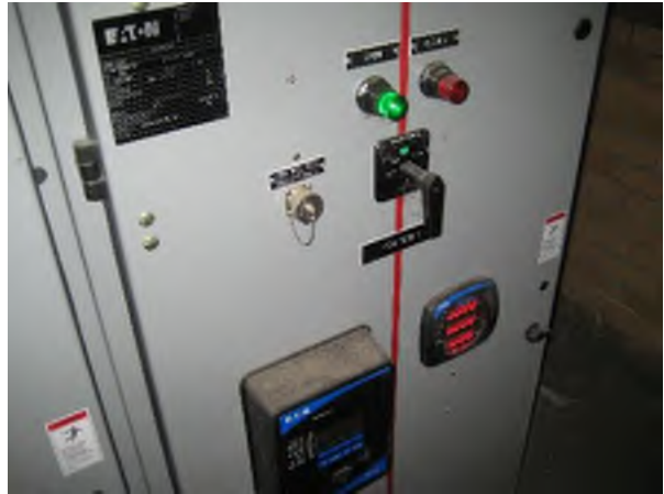
Main Switchgear Bucket Missing Arc Flash Label
