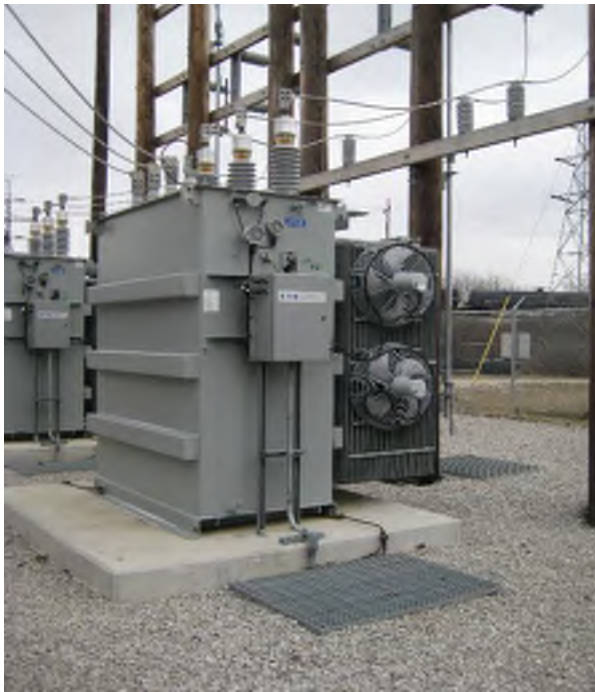
Plant-Owned 3500kVA, 46-k-2400V Transformers
