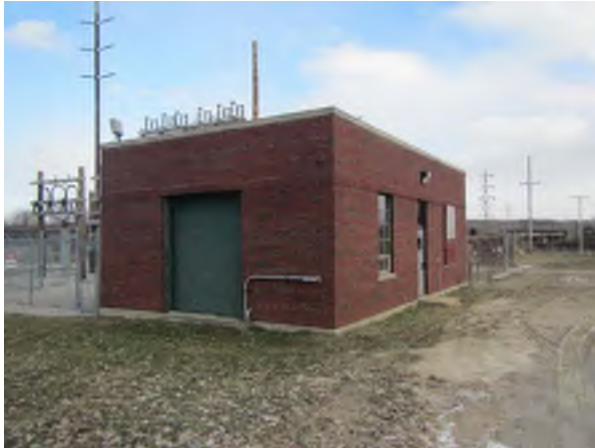
Northeast Electrical Building
