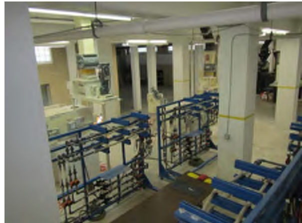
Ground Floor Level, Looking Southwest
