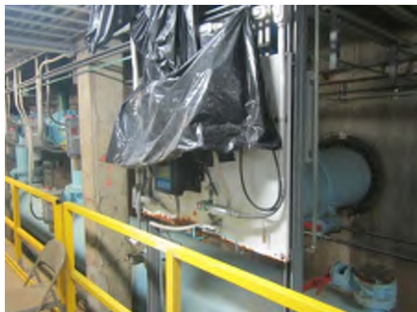
Plastic Bag Placed Over Control Panel
