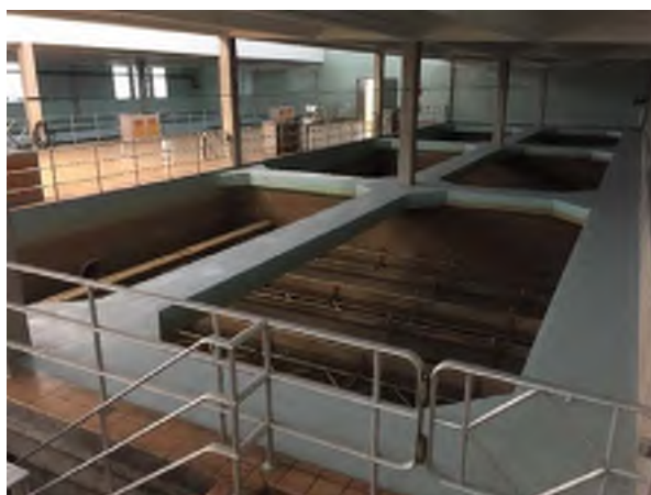
Existing Troughs for Media Filtration
