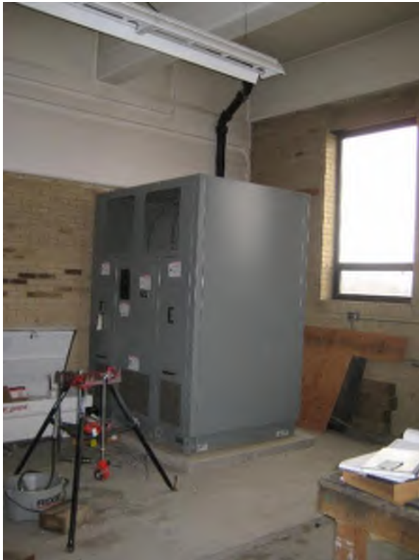
Single Transformer Feeding MCC-F1
