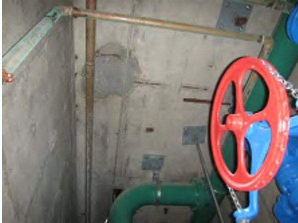
Previously Repaired Slab Spall, with Further Exposed Reinforcing Steel
