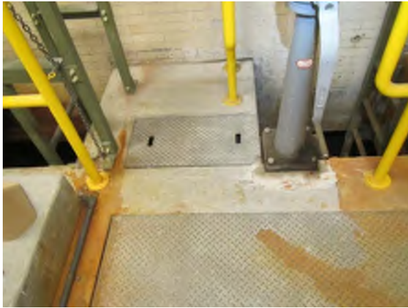
East Rapid Mixer Slide Gate, Cracked Operating Stand Anchorage
