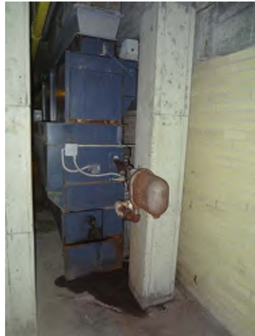
Heating and Ventilation System Serving Filter Gallery
