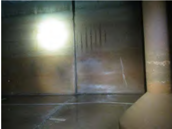
Corrosion of Vertical Wall Reinforcing
