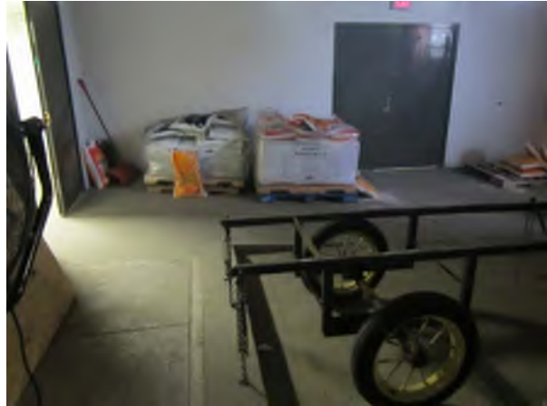
West Loading Area, Double-Leaf Hatch to Pipe Gallery
