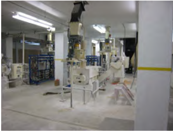
Lime Feed Area
