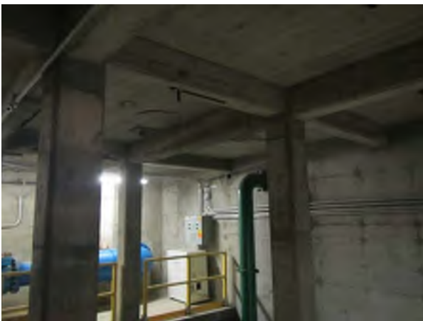
West Pipe Gallery Elevated Slab, Large Delamination about to Fall
