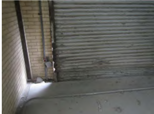
Corroded North Rollup Door Framing
