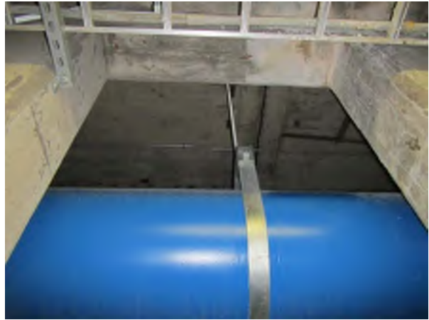
Corrosion Visible on Concrete Beam, Previously Completed Cementitious Repair
