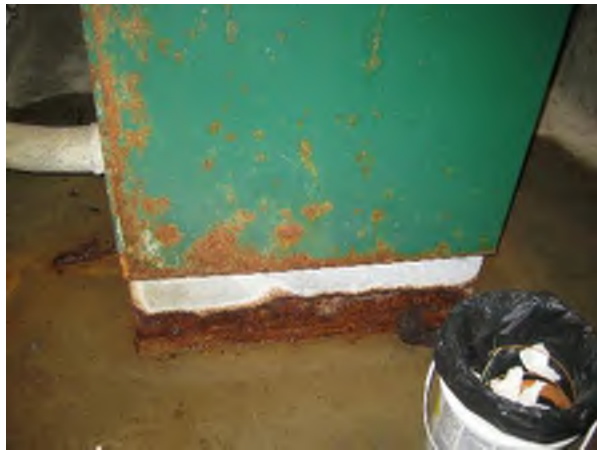
Kitchen Electrical Room 2400-480V/277V Transformer Disconnect Switch in Basement – Corroded Footings
