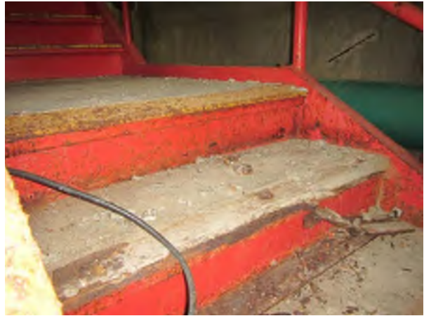
Lower Staircase Corrosion
