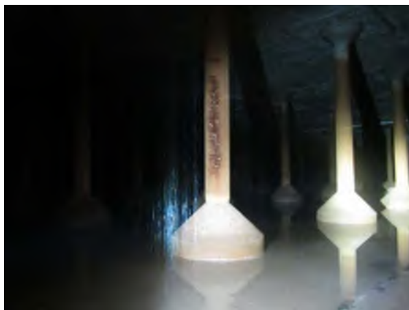
Column Deterioration and Corrosion, with Active Roof Leak at Expansion Joint
