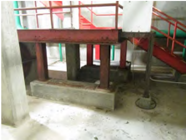
Lower Staircase, Corrosion Visible
