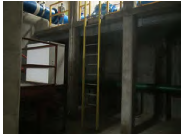
FRP Ladder Appears to be Missing Anchorage at Mid-Height
