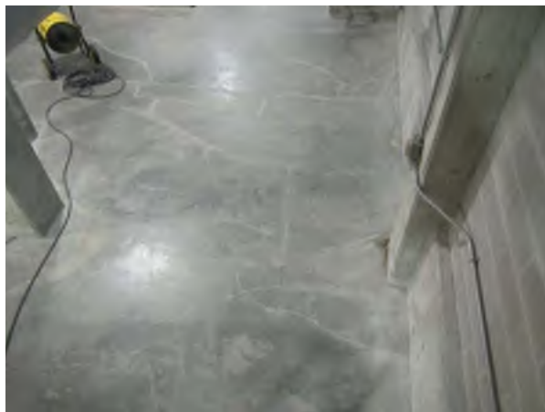
Elevated Floor Slab Cracking on Upper Level
