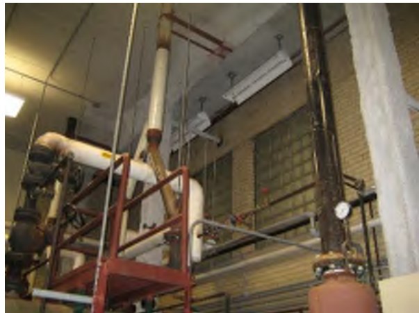
Luminaries that are not Easily Accessible Due to Height and Process Equipment
