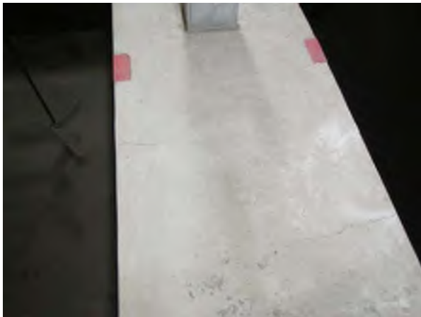
Cracked Elevated Walkway
