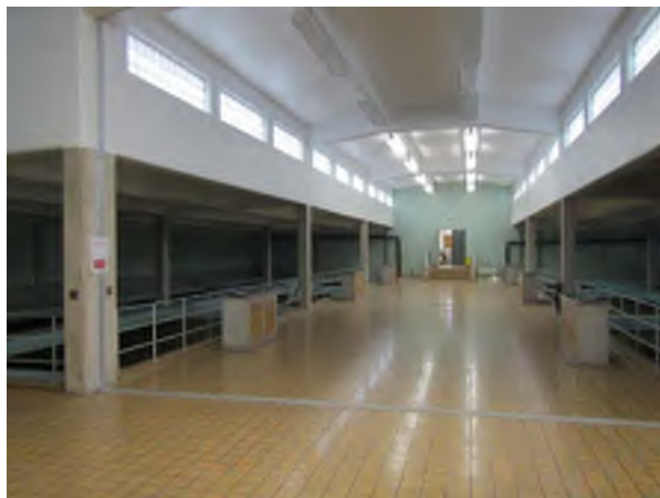
East Filters, Looking East
