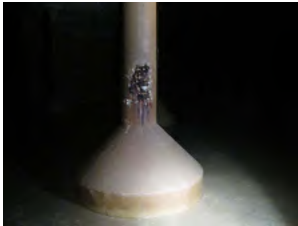
Column Deterioration and Corrosion
