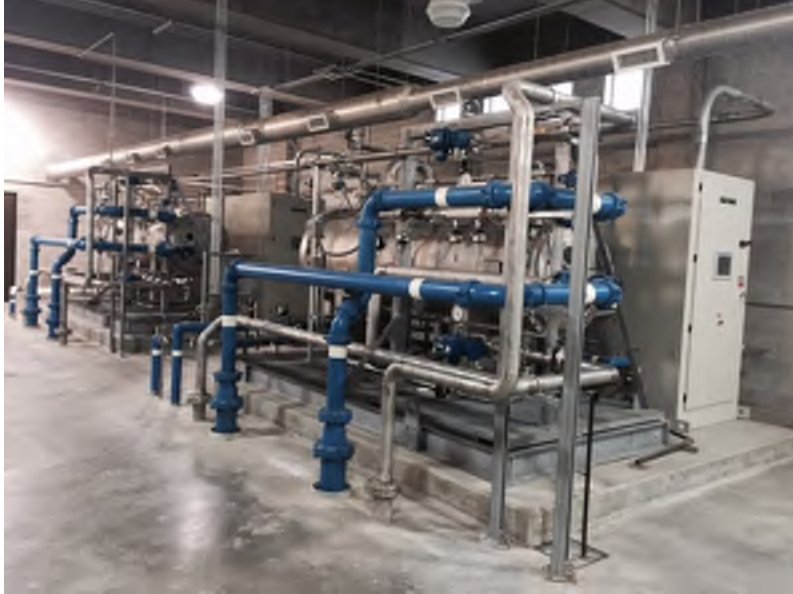
Figure 4.6 – Existing Ozone Generation Equipment for the Flint WTP
