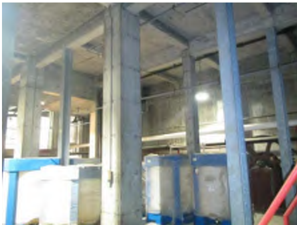
Additional Structural Columns in West Chemical Area Lower Level
