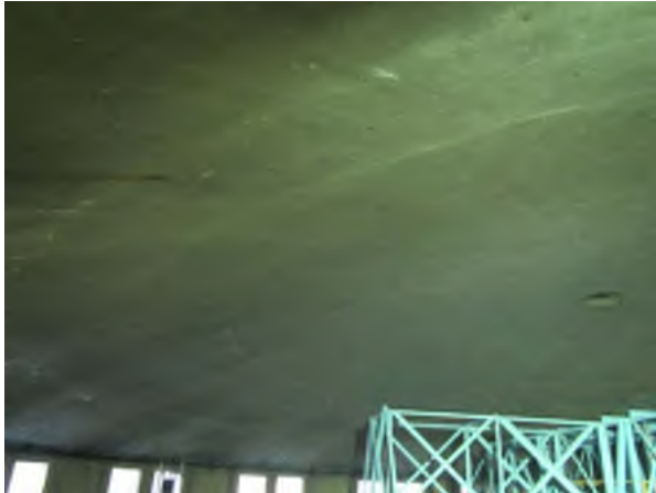
Old East Clarifier Dome
