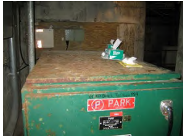
Kitchen Electrical Room 2400-480V/277V Transformer Disconnect Switch in Basement – Corroded Top of Enclosure
