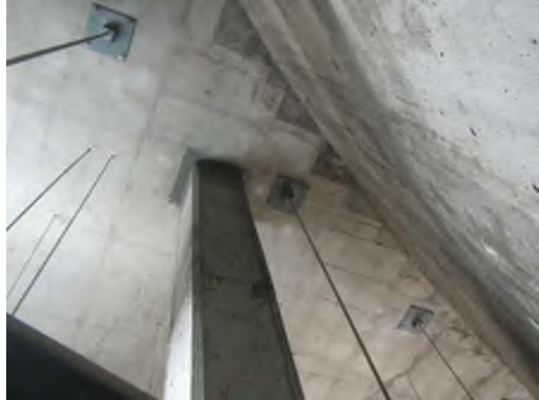
Cementitious Repair at Top Column, Lower Level, Corroded Rebar Chairs in Slab
