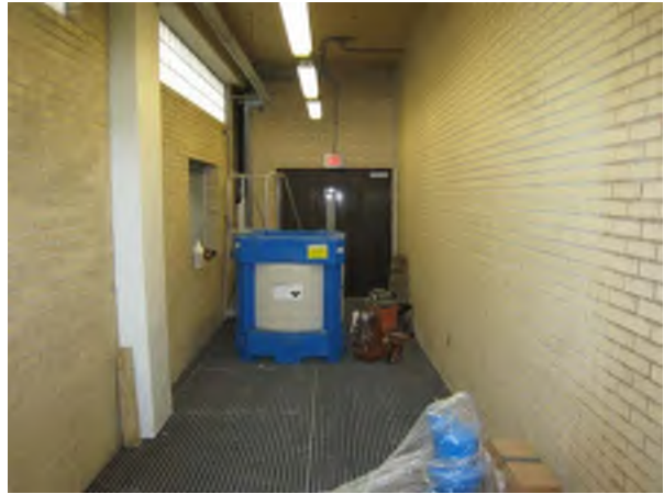
Chlorine Storage Room
