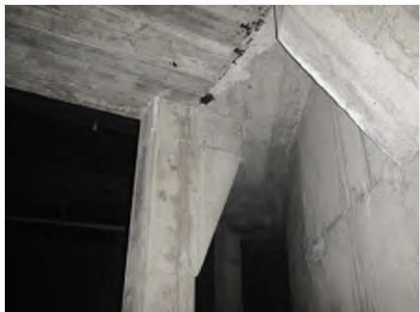
Shear Crack on Corbel with Slab Punching Shear Crack Visible
