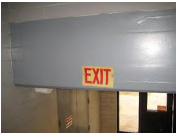
Improper Exit Sign
