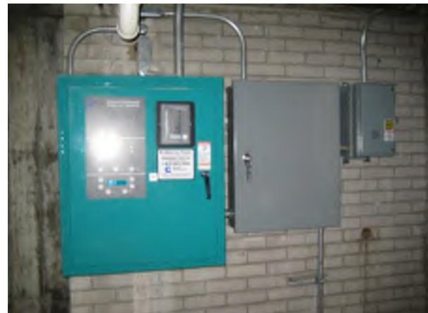
Generator Automatic Transfer Switch and Unlabeled Emergency Lighting Panelboard
