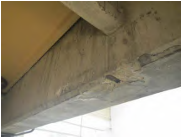
Beam Spalling
