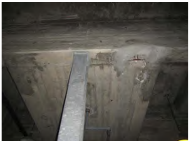
Additional Steel Column, Previous Concrete Repair, Exposed/Corroded Reinforcing Steel, West Chemical Area Lower Level
