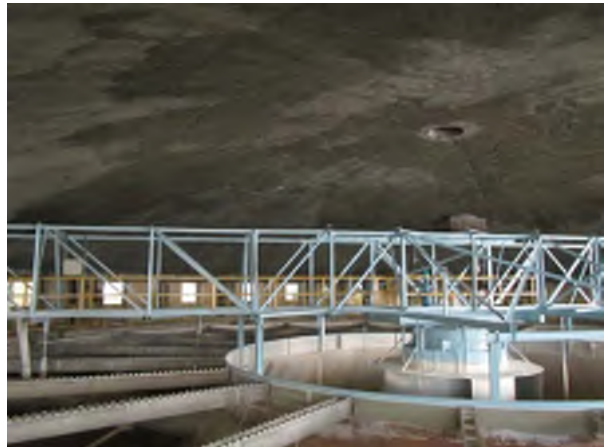
Old West Clarifier Dome
