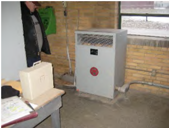
225kVA Transformer across the Main Switchgear
