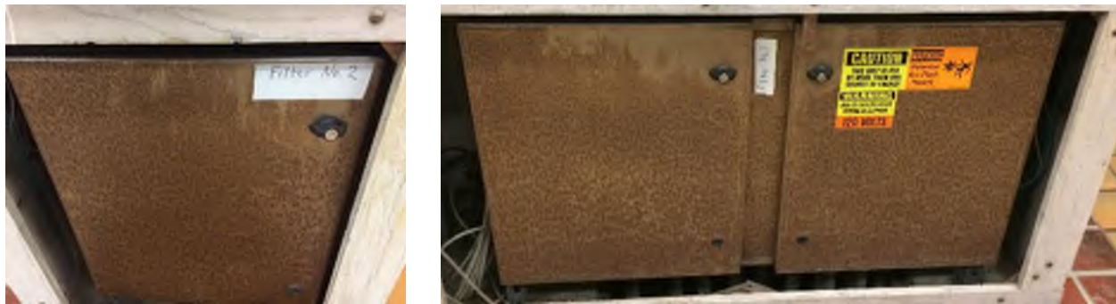
Filter Control Panel Enclosures
