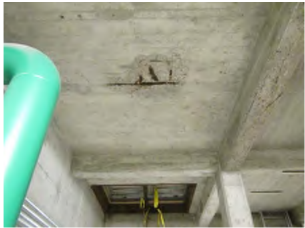
Underside of Elevated Slab, Beam Cracking/Delamination, Slab Spalling
