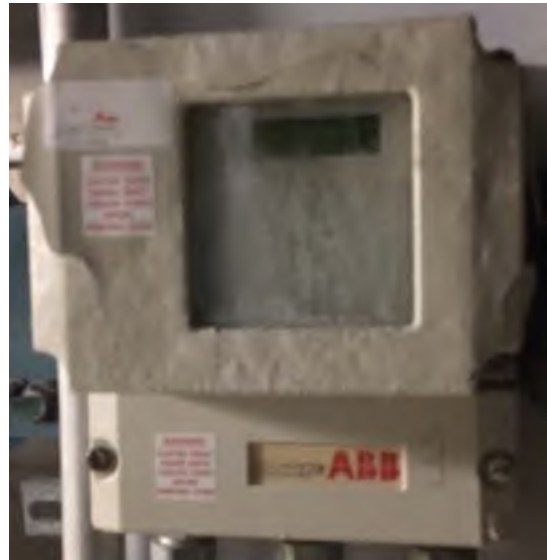
Filter No. 3 Damaged Flow Transmitter
