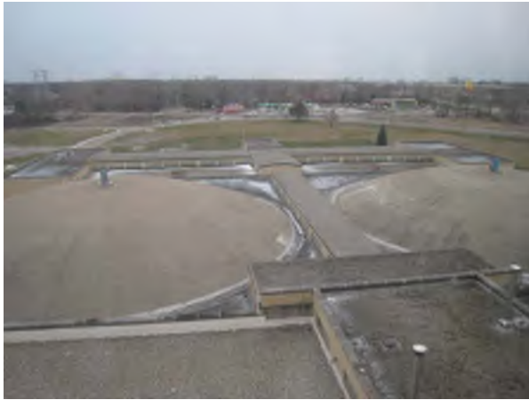
Roof Looking South
