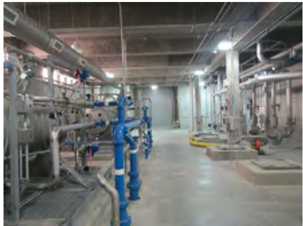
Upper Level, Looking South
