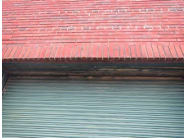
Northeast Electrical Building, West Rollup Door Lintel Deflection
