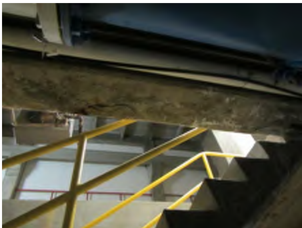
East Loading Area Concrete Beam Delamination
