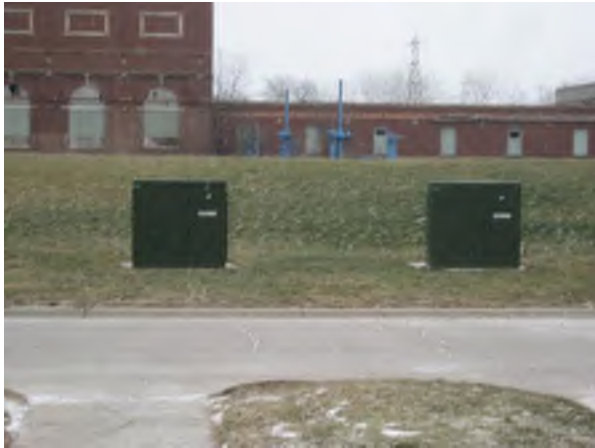
Plant #2 – 2400-480V Transformers
