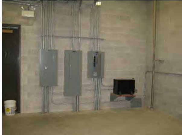
Panelboards and UPS
