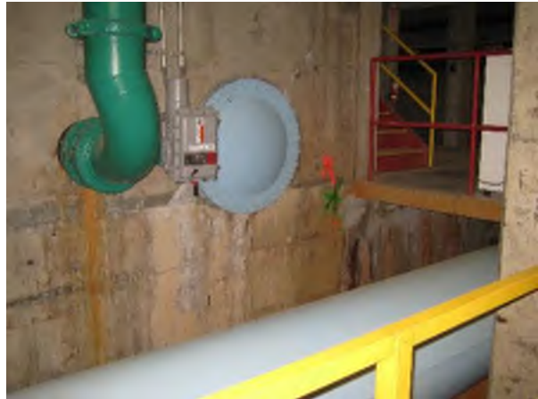
Valve Control Panel Located in Pipe Gallery without Ease of Access for Manual Controls
