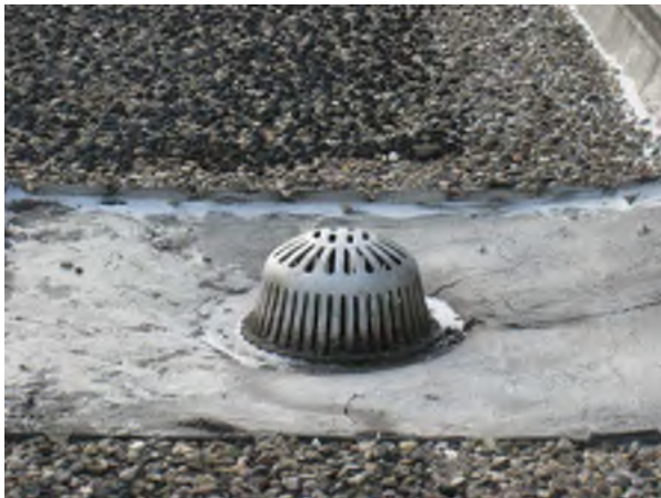
Typical Roof Drain
