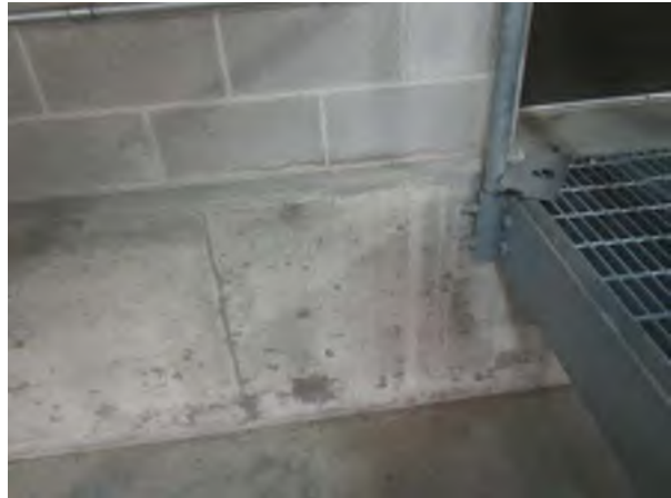
West Perimeter Upper Level Beam Cracking
