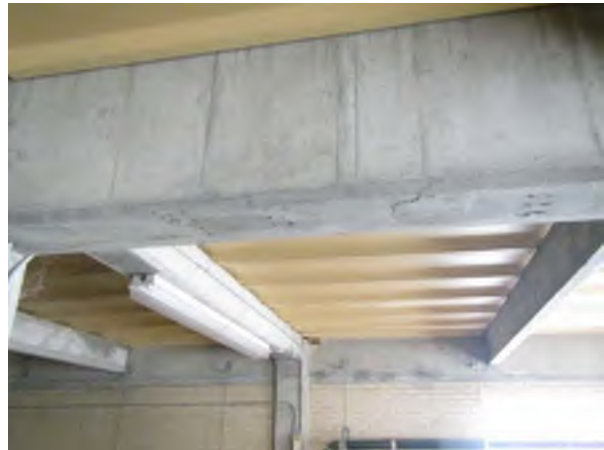
Beam Delamination, Visible Corroded Rebar Chairs
