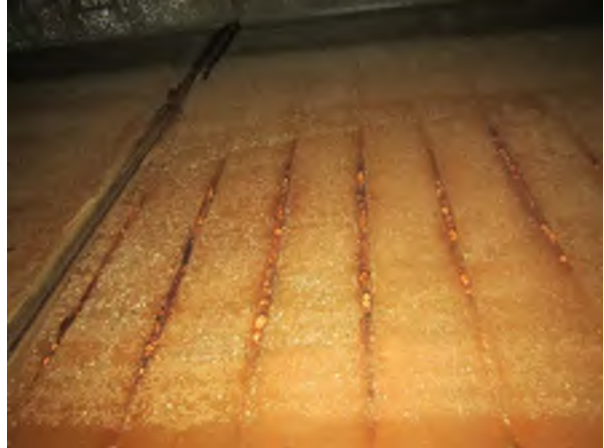
Corrosion of Vertical Wall Reinforcing
