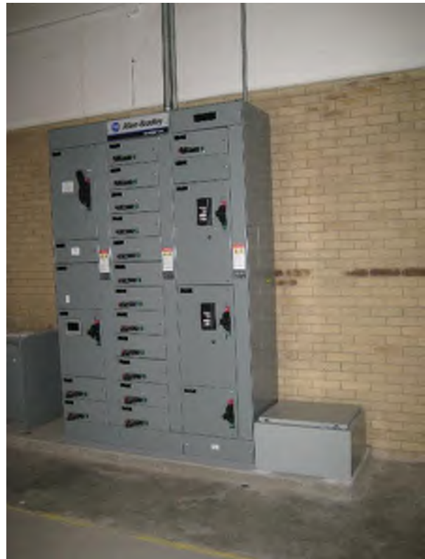
Old B&G Motor Control Center (MCC-F1)
