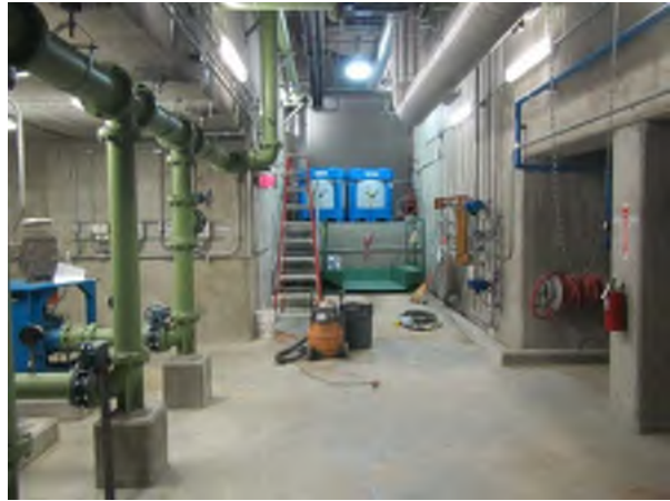
Ozone Building, Lower Level Gallery
