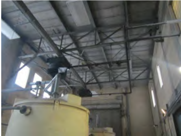
West Loading Building, Looking North
