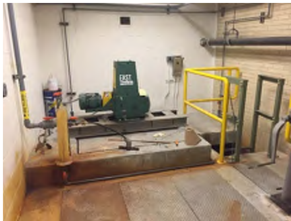
Existing Rapid Mixer Equipment
