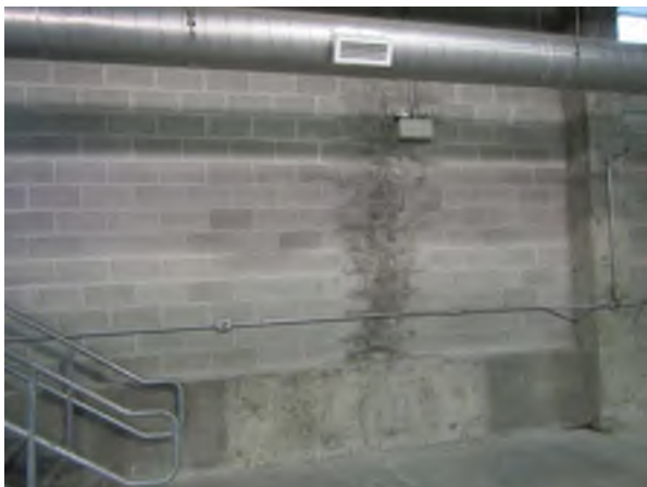
West Exterior Masonry Wall Discoloration, Upper Level
