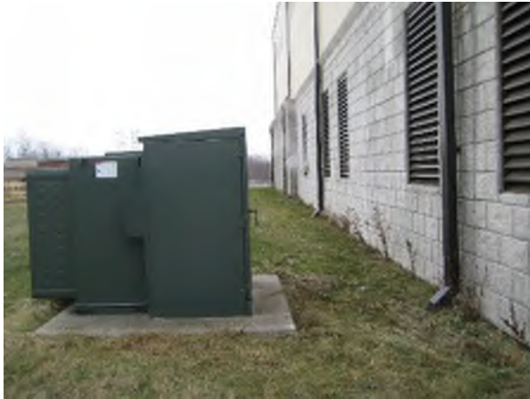
Single Transformer Feeding the Ozone Building
