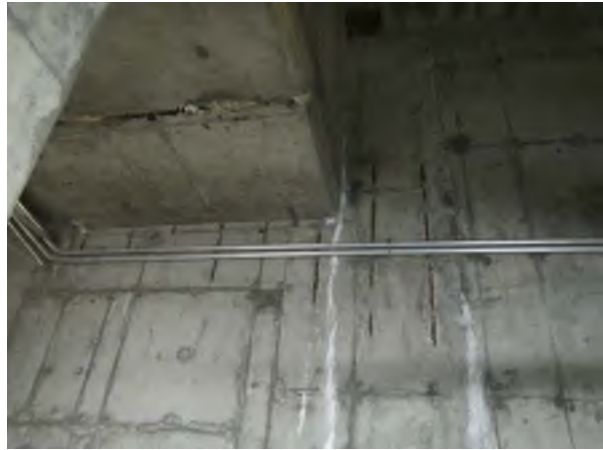
Exposed Vertical Wall Reinforcing
