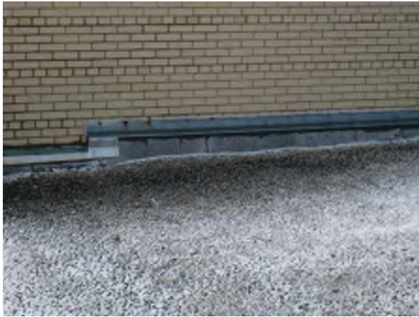
Typical Counterflashing
