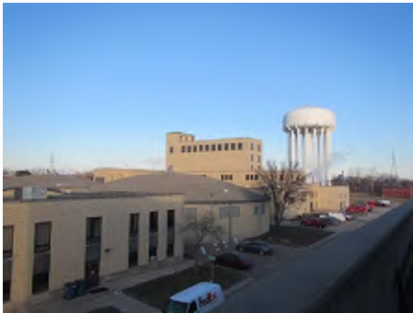
Exterior of East Clarifier
