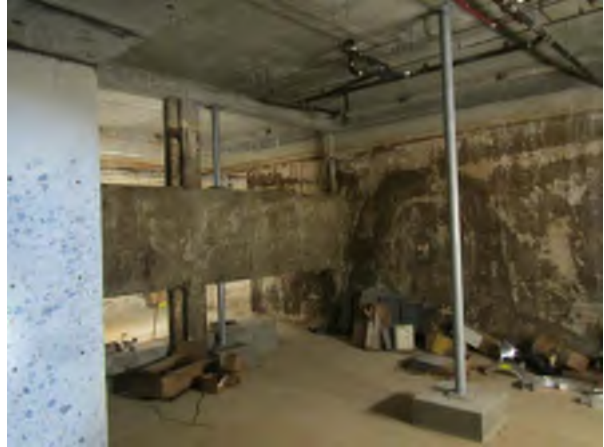
East Old Slow Mix Tank, Additional Steel Columns
