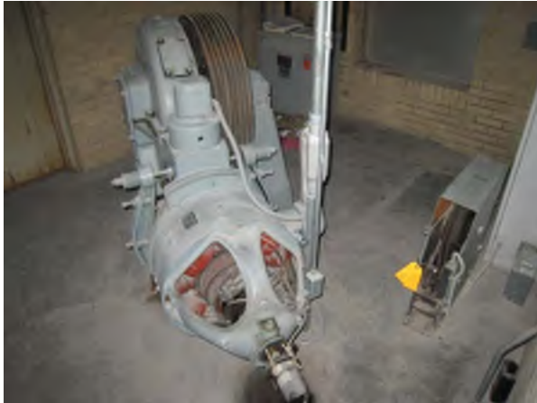
Elevator Equipment Room
