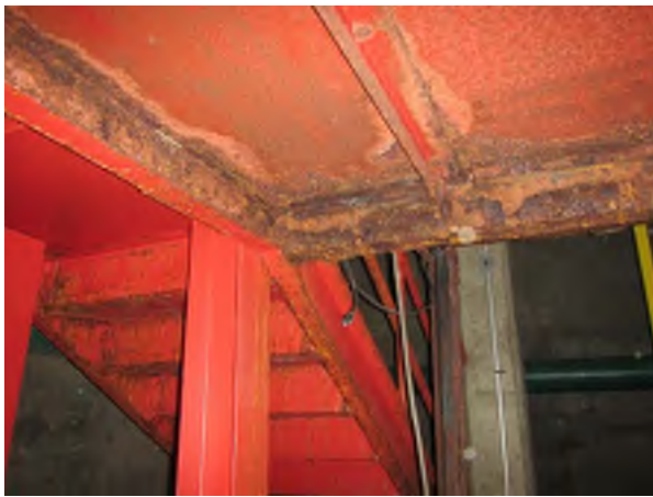
Lower Staircase Corrosion
