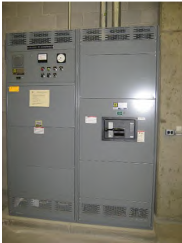
MCC-OZ External Main Circuit Breaker
