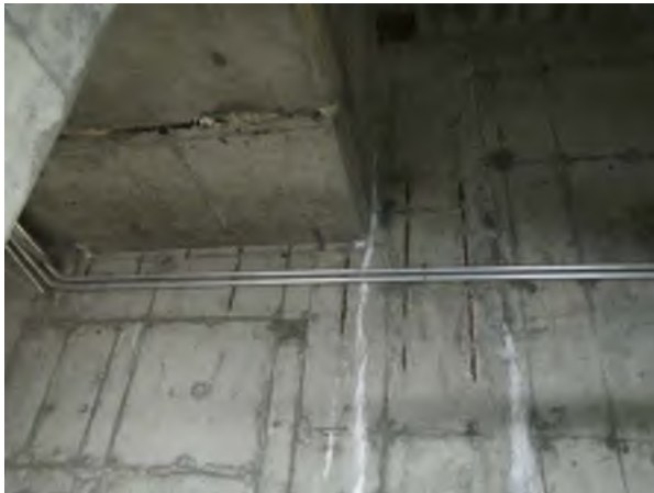
Exposed Vertical Wall Reinforcing
