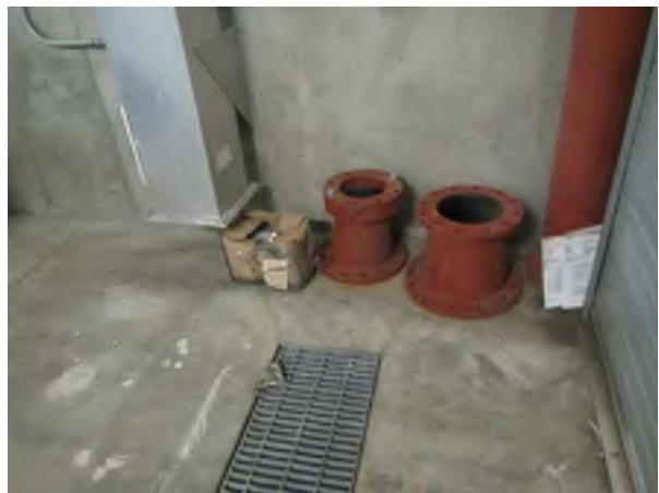
Trench Drain Cracking at Re-Entrant Corners
