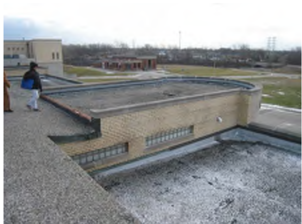
Roof and Drain at South Entry
