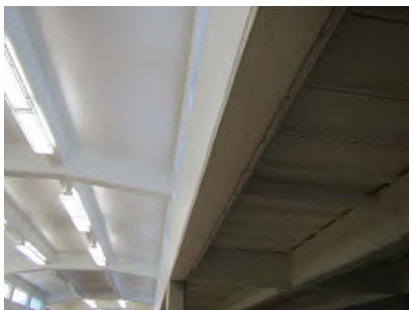
Rebar Chair Corrosion, Visible through Paint
