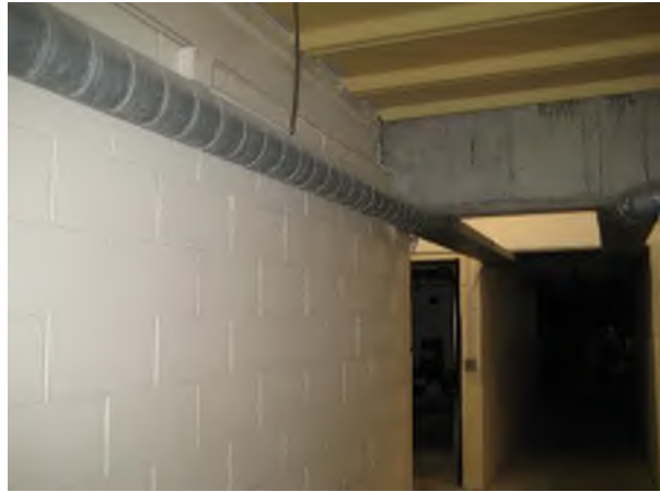
Floc Mixer/Clarifier Hallway with Inadequate Emergency Lighting & Exit Signs
