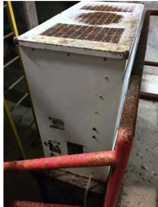
Portable Dehumidification Units in Pipe Gallery
