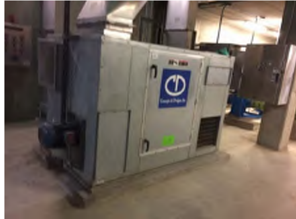
Dehumidification Air Handling Units at Ozone Building
