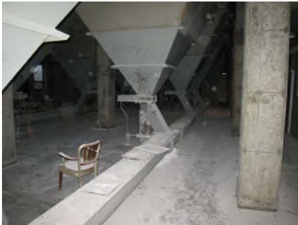
Lime Storage Area
