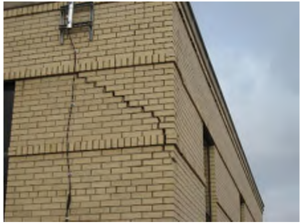
Cracks at the Corner of Lime Area
