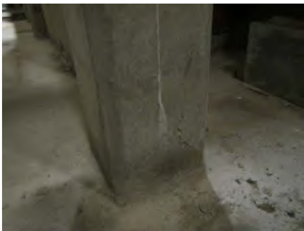
Column Cracking at Base
