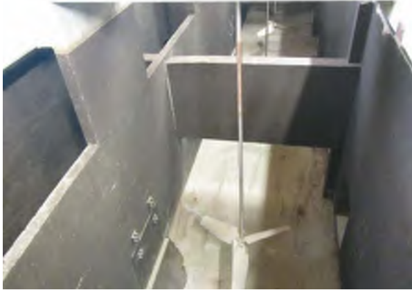
Flocculation Tank Interior, typical
