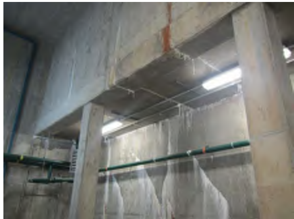
West Wall, Visible Cracking, Looking East
