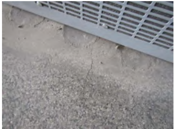
Floor Crack at Penetration
