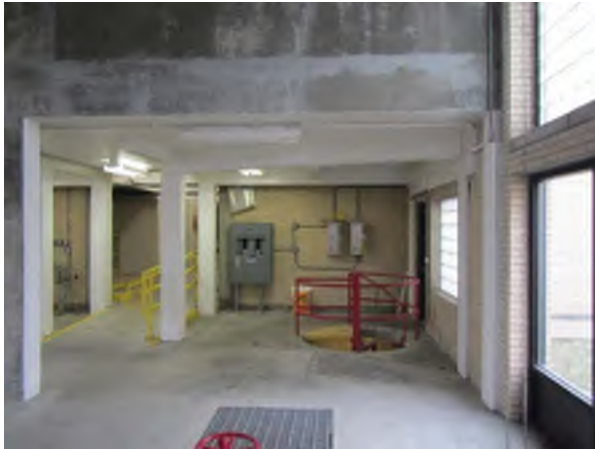
IPS Connection, Ground Level, Looking South
