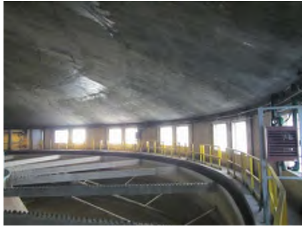
Old West Clarifier
