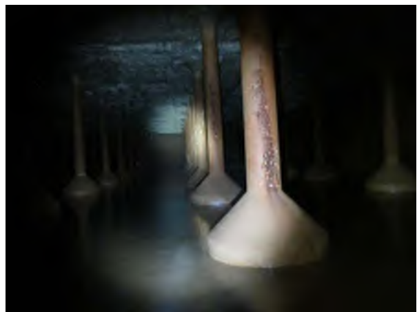
Column Deterioration and Corrosion
