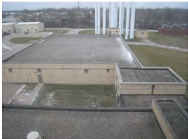
Roof at Clarifier Area
