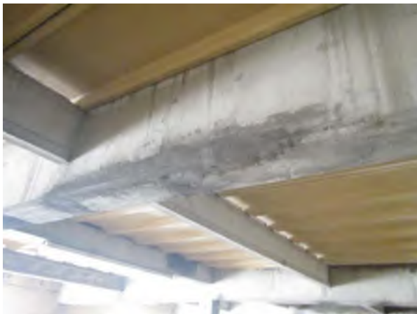
Beam Repair in West Flocculation Room
