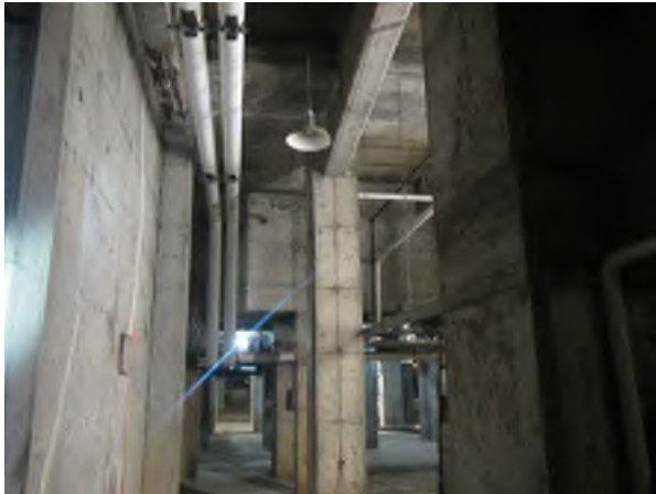
Beam Spalling and Exposed/Corroded Rebar in East Chemical Area
