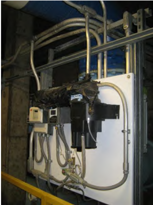
Instruments in Filter Pipe Gallery Below Leaking Process Pipes
