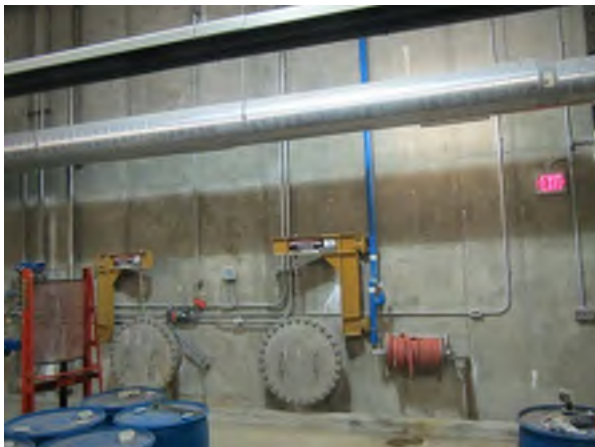
Interior Tank Wall
