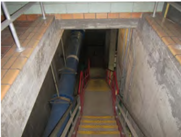
Staircase Down to West Pipe Gallery
