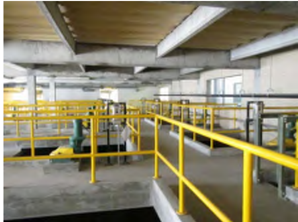
West Flocculation Room
