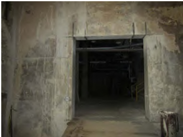
East Old Slow Mix Chamber, Square Penetration
