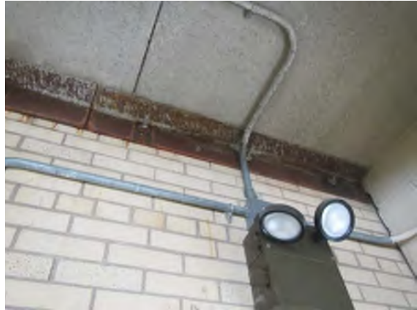
Roof Plank Shelf Angles
