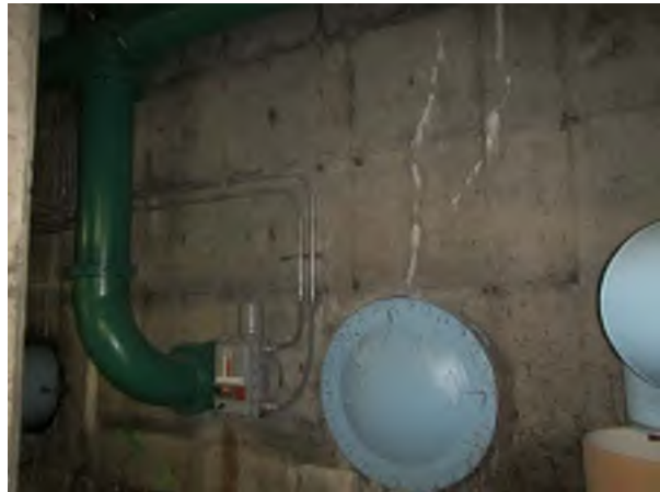
Wall Cracking
