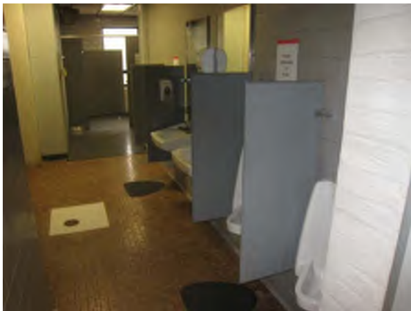
Men's Locker Room
