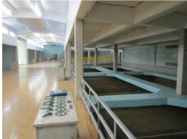
Rapid Sand Filter Building, Operating Floor, Looking West
