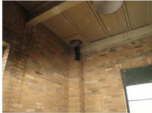
Ceiling and Roof Drain
