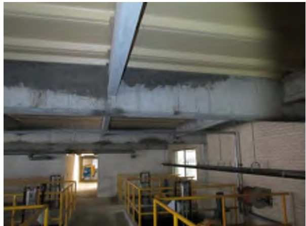
Beam Repair in West Flocculation Room
