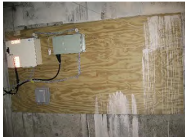
Telephone Backboard in Basement Below Kitchen Electrical Room
