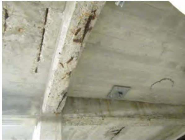
Underside of Elevated Slab, Concrete Deterioration, Spalling, Exposed/Corroded Rebar, Delamination
