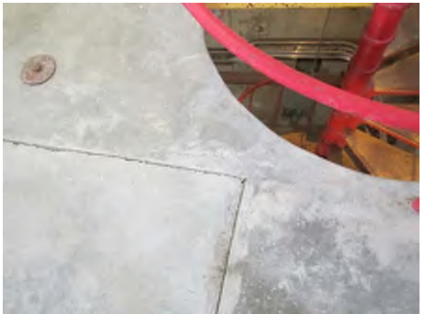
Slab Cracking Adjacent to Spiral Staircase
