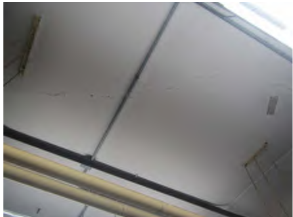
Outlet Structure Slab Cracking
