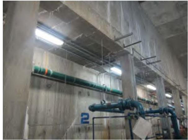
West Wall, Visible Cracking, Looking East
