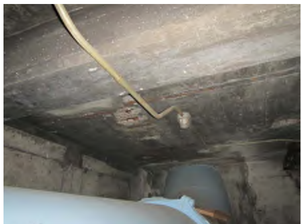
East Loading Area Slab Spall and Exposed Rebar
