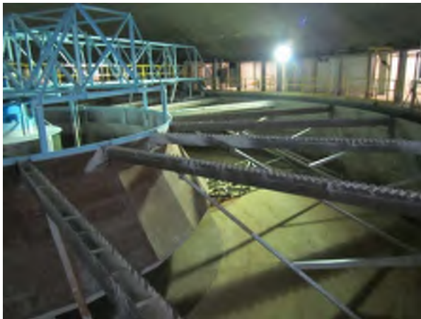
Old East Clarifier
