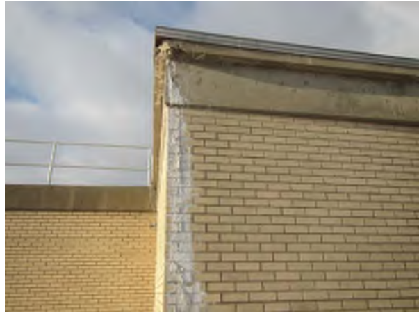
Inlet Structure Exterior Wall Cracking
