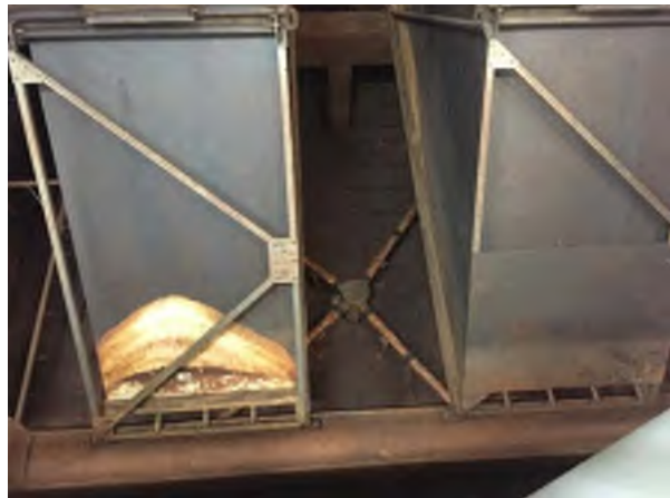
Existing Plate Settlers and Sludge Collection System
