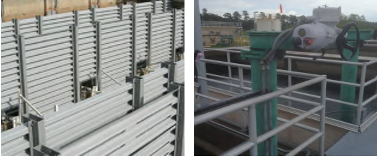
Figure 4.14 – Structural FRP Panel (by Enduro) and Torque Tube Operator Installed in a Flocculation Basin
