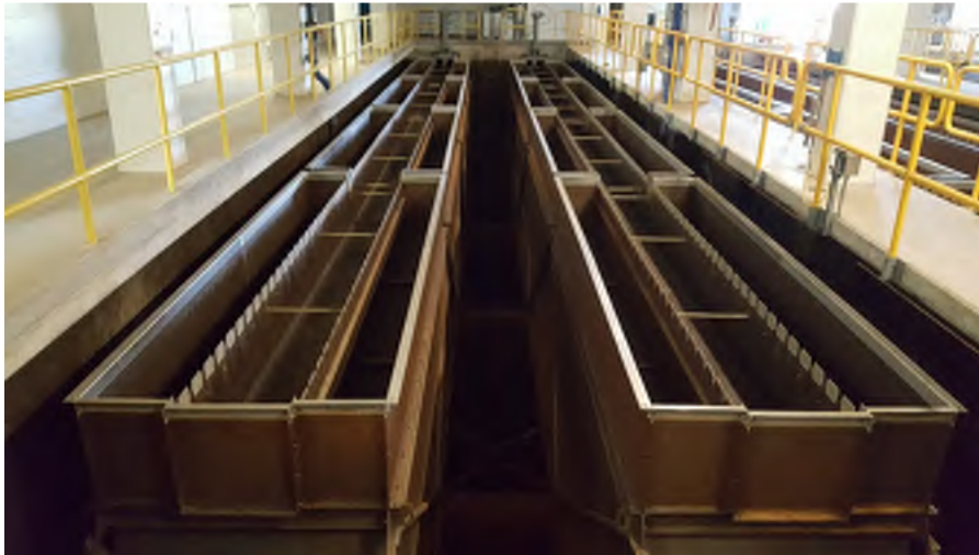
Figure 4.17 – Inclined Plate Settler Packs in Basin No. 1
