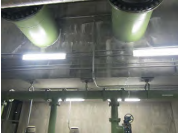
Cracking at Pipe Penetrations
