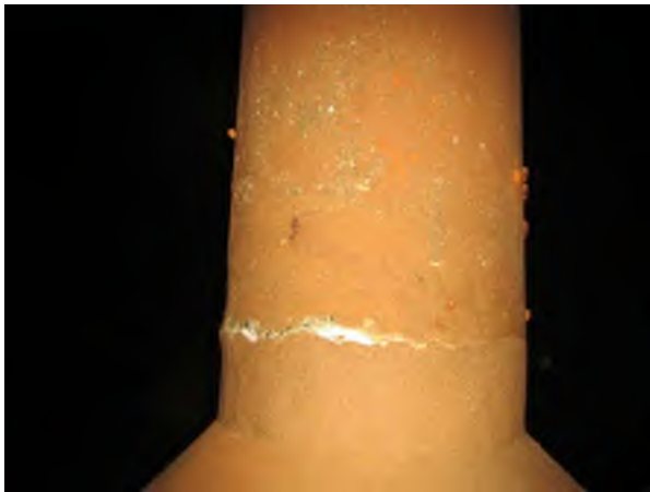
Circumferential Crack and Bulging near Column Pedestal
