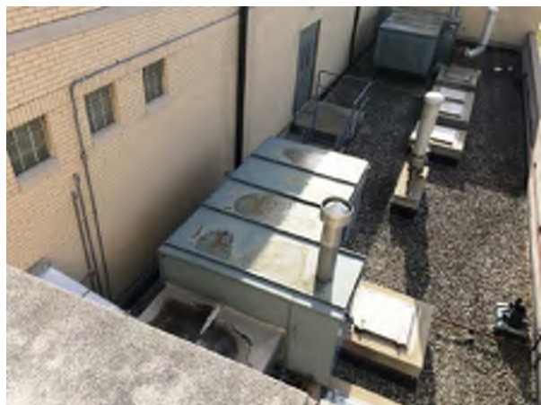
Rooftop Makeup Air Units
