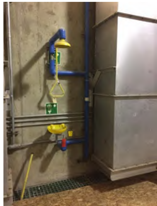
Emergency Shower/Eyewash in Ozone Building
