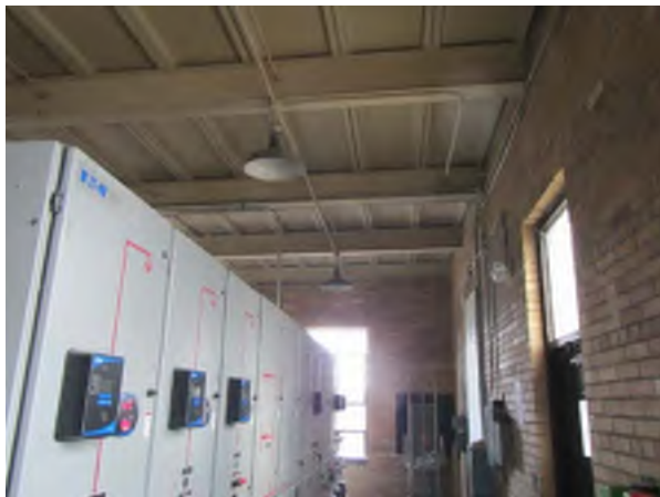
Northeast Electrical Building, Looking East
