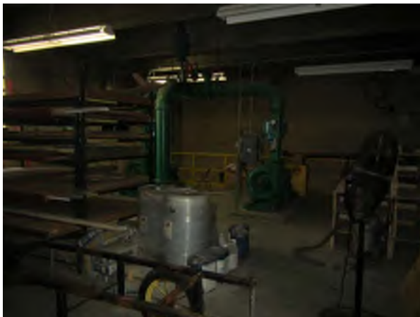
West Loading Area, Blowers
