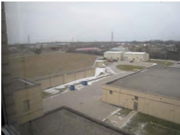
Roof at Clarifier Addition
