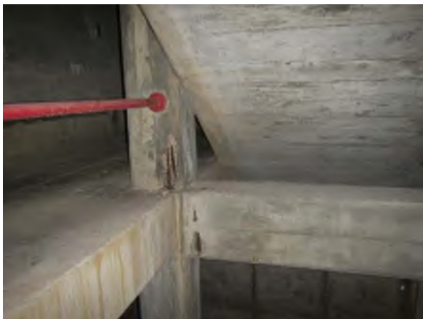
East Loading Area Column and Beam Spall, Exposed Rebar
