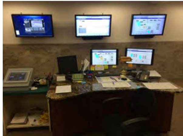
Control Room Console
