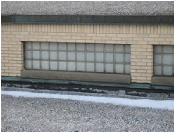
Typical Glass Block Window
