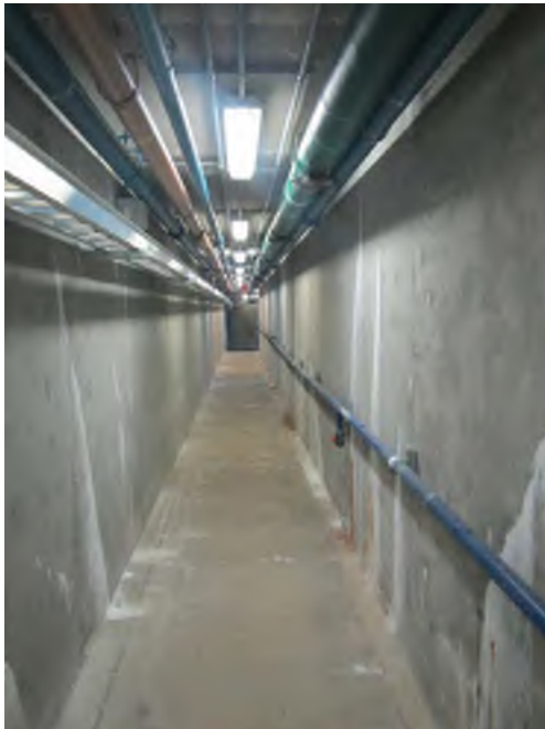
Wall and Slab Cracking in Lower Level, South Corridor
