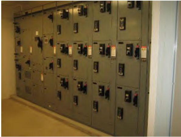
MCC-1 (West Floc Mixer Control Room)
