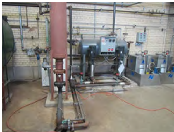
Boiler Building, Looking West
