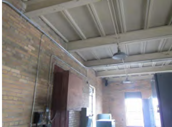
Northeast Electrical Building
