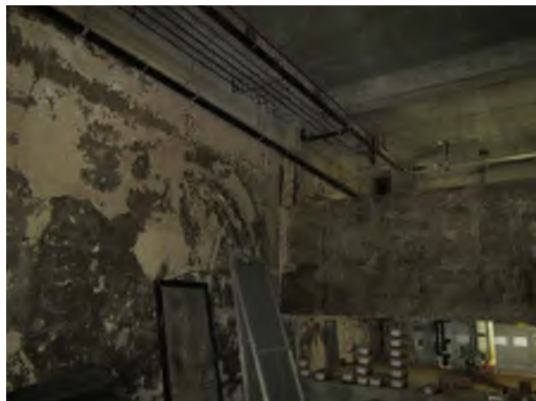
Modification to Original Structure, New Beams and Slab
