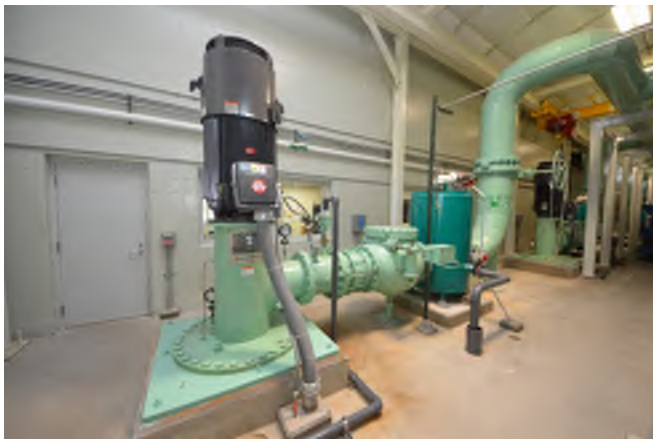
Figure 6.2 – Vertical Turbine Pump
