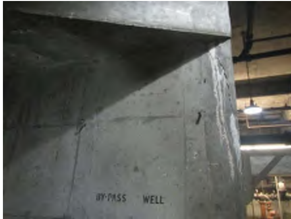
Bypass Well Cracking, Chemical Area Lower Level
