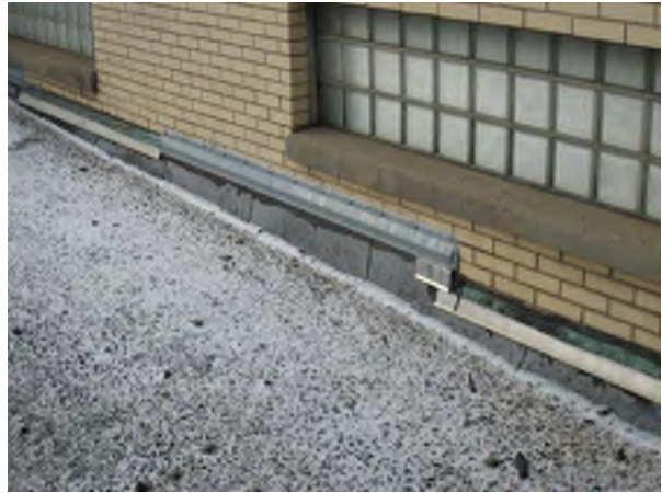
Typical Counterflashing
