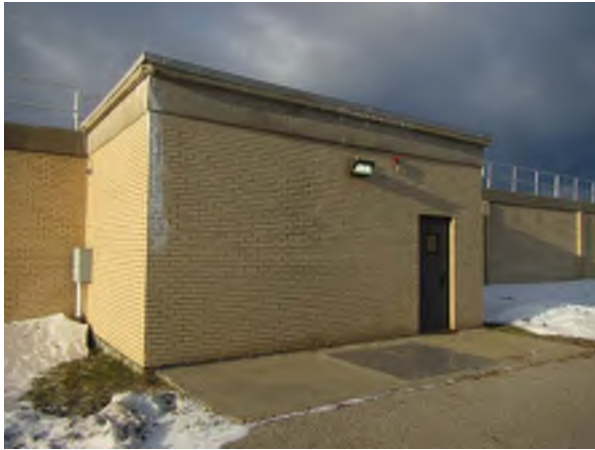
Inlet Structure Exterior
