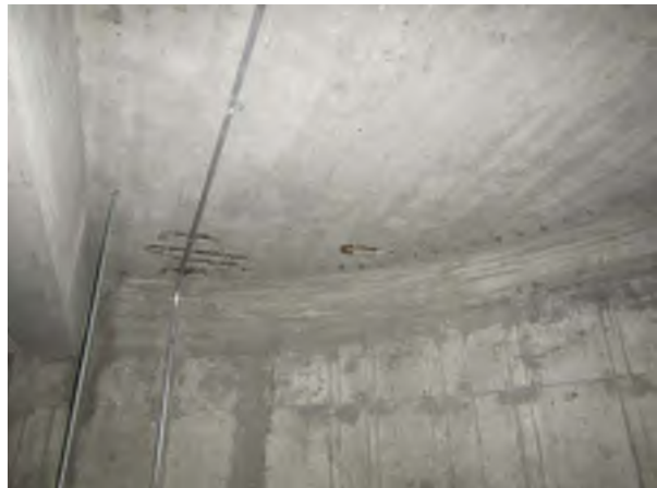
Main Entrance, Underside of Elevated Slab, Exposed/Corroded Rebar, Visible Rebar Chair Corrosion
