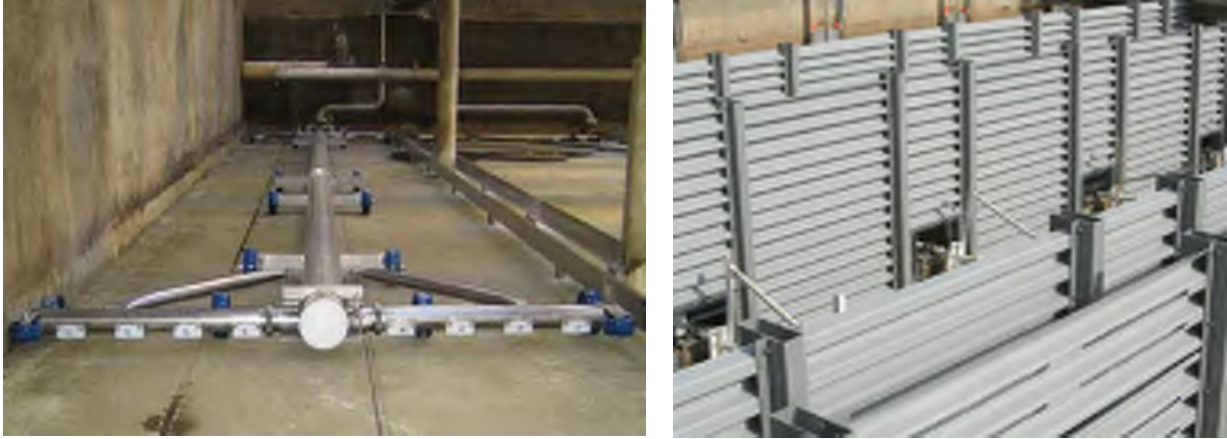
Figure 4.18 – MRI Hoseless Cablevac Sludge Collector System (by Meurer Research) and FRP Baffle Wall (by Enduro)
