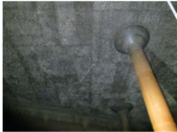
Roof Slab Crack from Column Drop Panel to West Exterior Wall of Area #6
