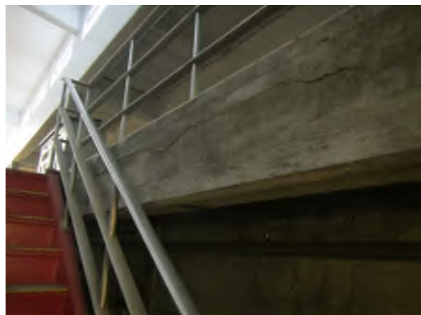
Beam Cracking and Delamination at West Staircase
