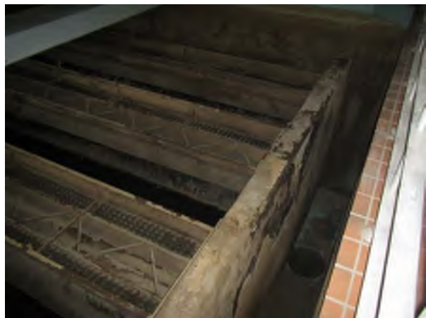
Filter Box, Minor Discoloration but no Visible Cracking
