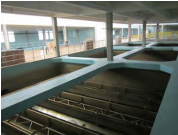
East Filters, Looking Southwest
