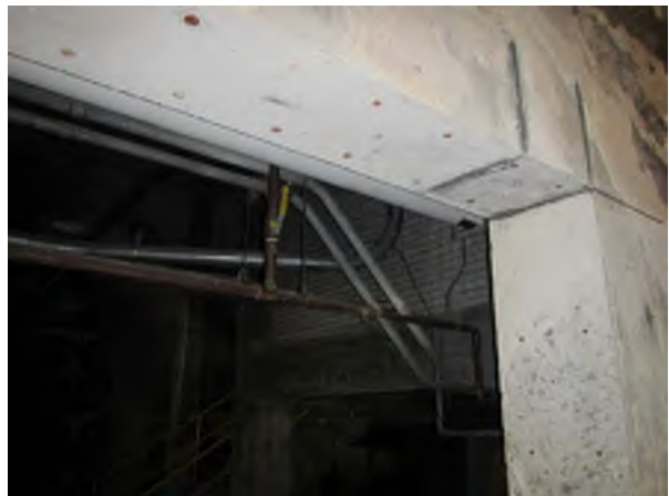
Exposed Rebar Ends from Saw Cutting
