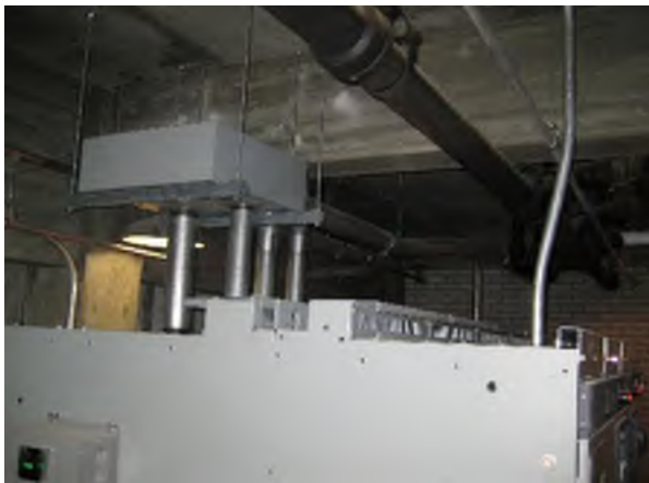
Locker Room Sanitation Line Directly Above Switchgear
