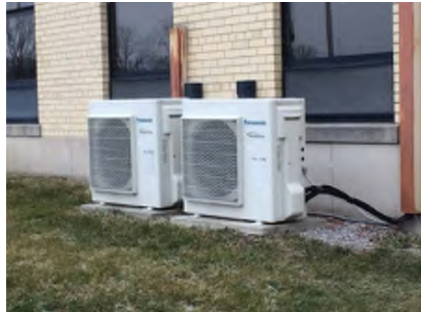
Front Office Split System Units
