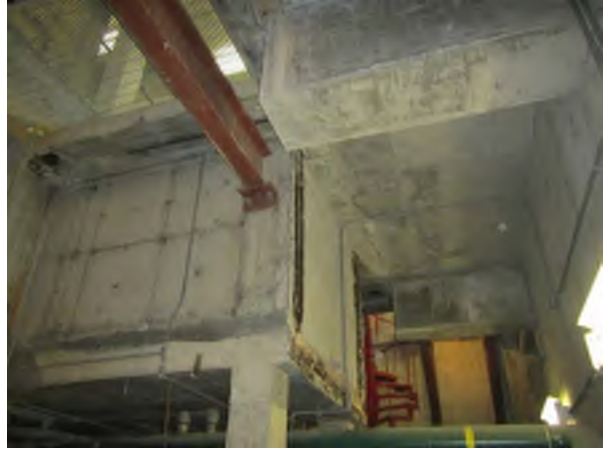
IPS Connection, Lower Level, Looking West, Local Spalling/Corrosion in Cantilevered Slab to East of Water Conduit
