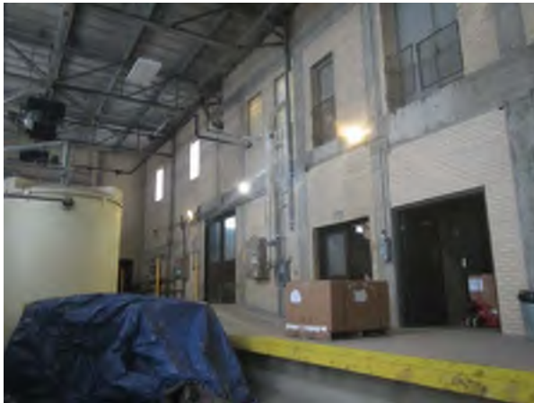
West Loading Building, Looking Northeast
