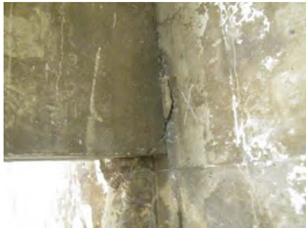
East Old Slow Mix, Crack at Weir Wall Support
