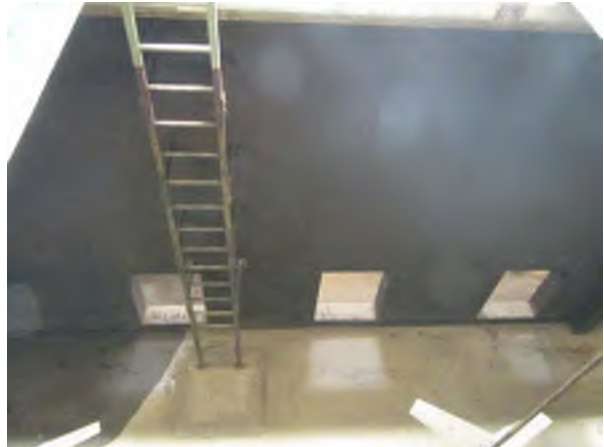
Flocculation Tank Interior, typical
