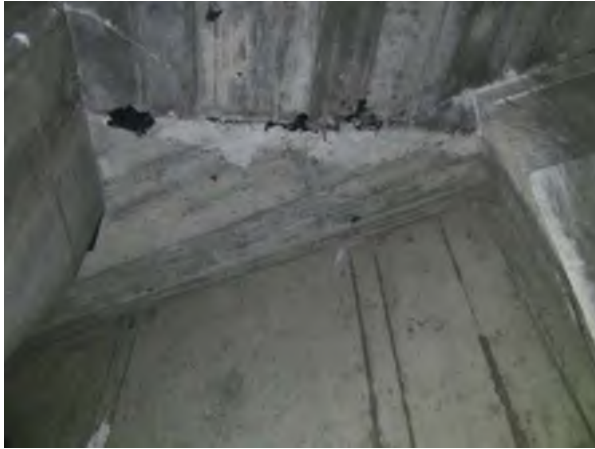
Punching Shear Crack
