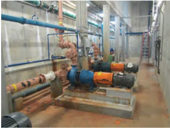
West Wall, Visible Cracking, Looking Southeast
