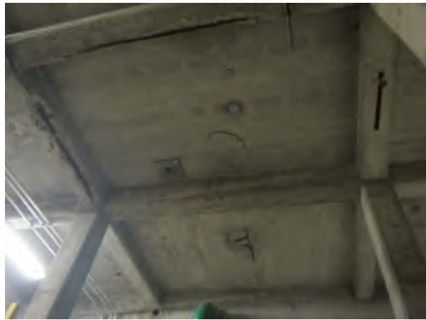
Elevated Slab, Visible Delamination, Exposed/Corroded Rebar
