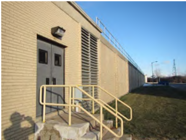
Outlet Structure Exterior
