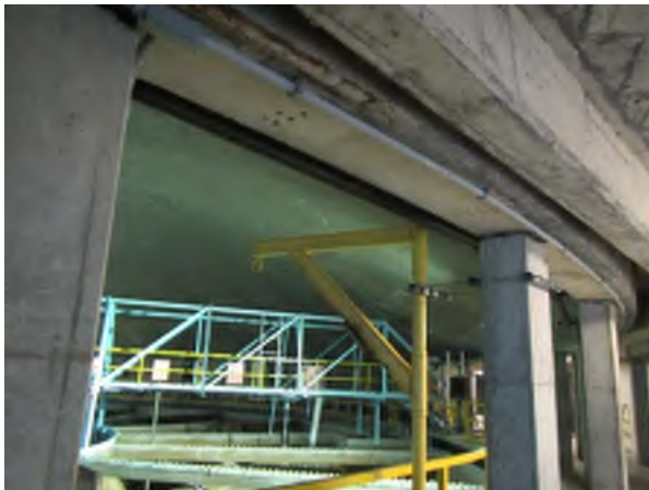
Ring Beam Corrosion and Delamination, Corroded Rebar Chairs Visible
