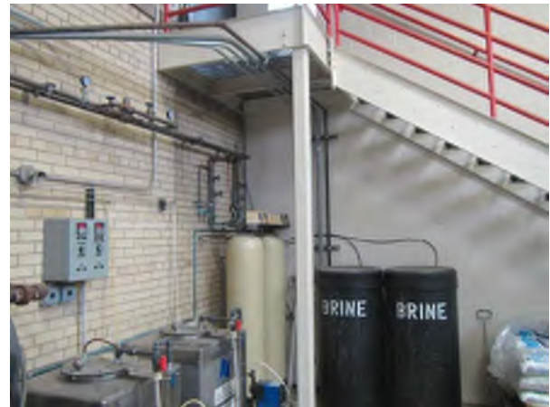
Boiler Building Staircase
