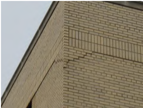
Cracks at the Corner of Lime Area
