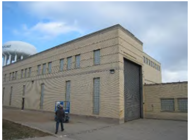
Cracks at Corner by Door
