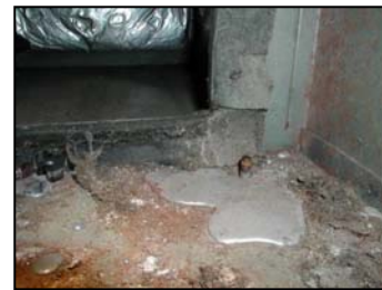
Mercury at the bottom of the return-air duct in a furnace
