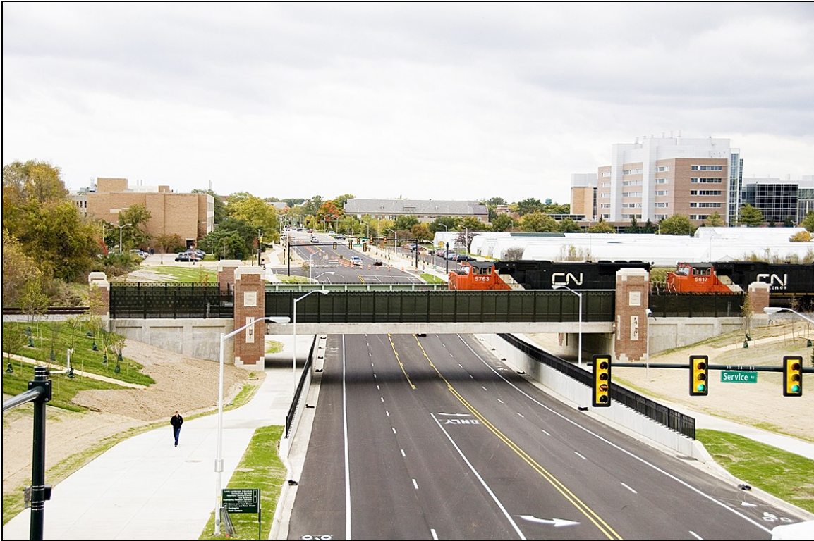
Figure 4 Grade Separation Underpass with Sidewalk and Bike Lanes on Michigan State University Campus
