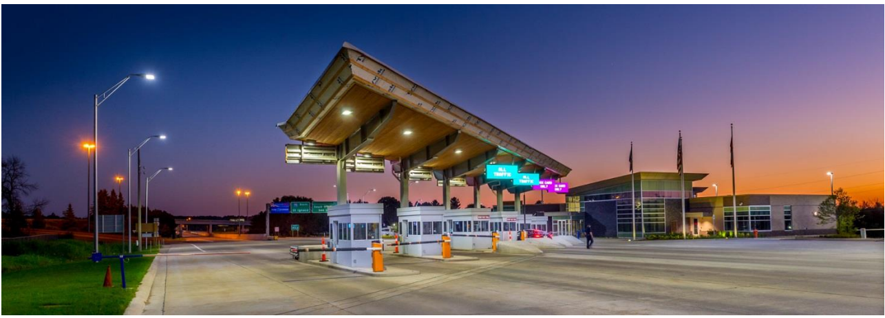
The award-winning Sault Ste. Marie International Bridge toll plaza project shown as it was nearing completion. (MDOT Photo)
