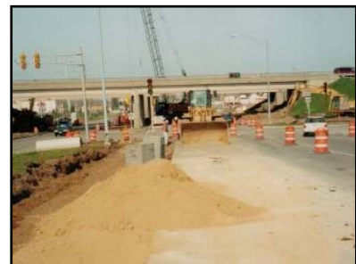
MDOT will develop plans to keep traffic moving during construction.
