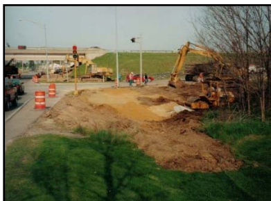
Construction activities would have temporary visual impacts.
