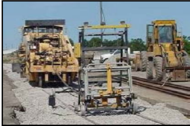
Construction equipment would generate temporary noise impacts.
