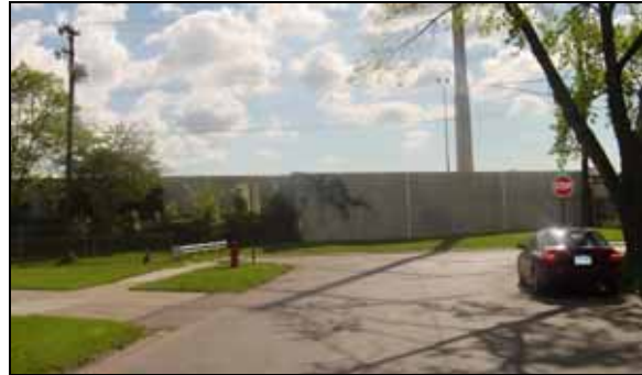
Example of Security Wall in Residential Area at Nearby Melvindale Terminal
