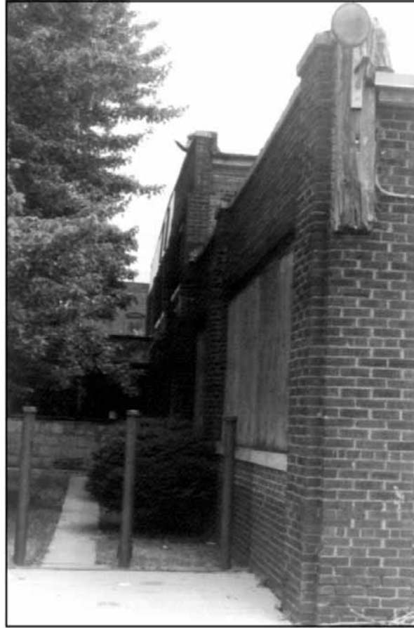
Michigan Box Company — North Wall, View to East.
