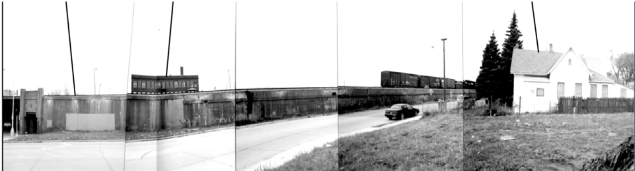
6332 John Kronk Streetscape, View to south-southwest toward rail yard from house (house is on the right)
