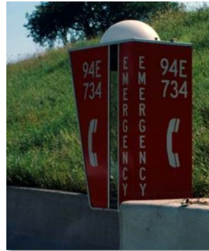
Figure 4. A motorist-aid telephone. (Source: A History of ITS in Detroit, SEMTOC.)
