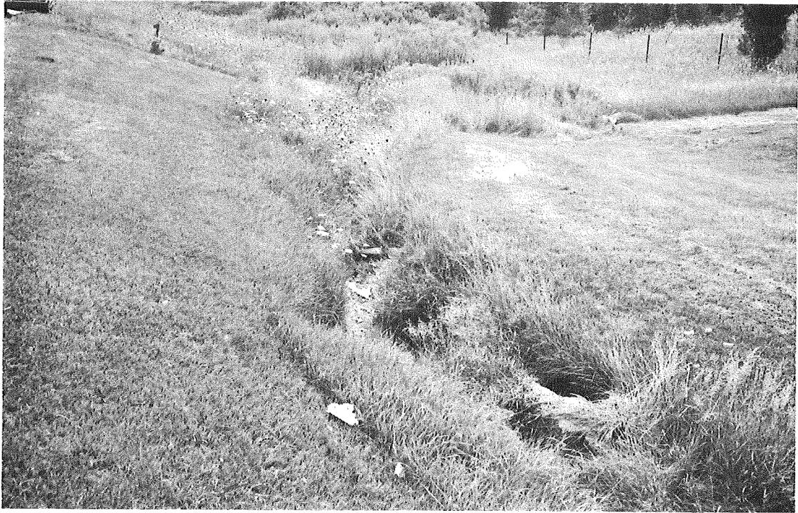
Figure 3. Erosion problems at the Novi rest area drainage ditch.
