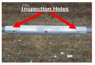
**NOTE:** Check both inspection holes while loosening turnbuckle.
