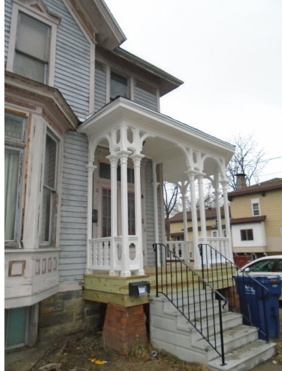
HDF-2017-5836-NEP, 521 N. Grant St., Porch Repairs AFTER
