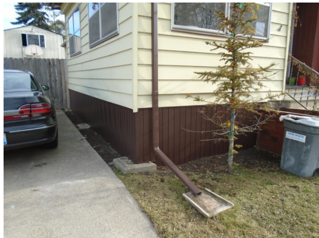
HDF-2017-5836-NEP, 510 N. Grant St., Porch Repairs AFTER
