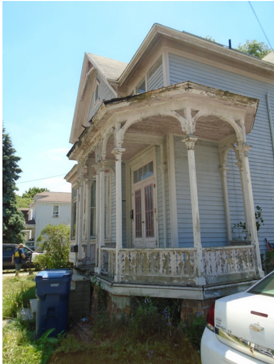
HDF-2017-5836-NEP, 521 N. Grant St., Porch Repairs BEFORE
