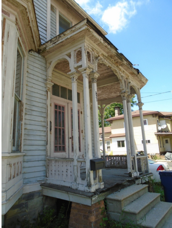
HDF-2017-5836-NEP, 521 N. Grant St., Porch Repairs BEFORE
