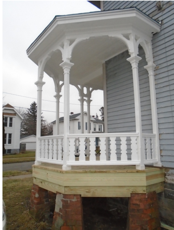
HDF-2017-5836-NEP, 521 N. Grant St., Porch Repairs AFTER
