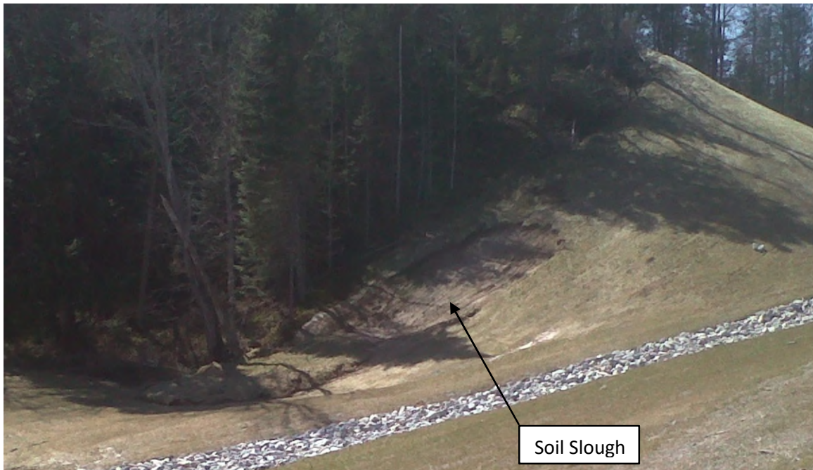
Figure 15: Soil Slough in Spring
