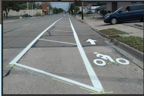
A **buffered bicycle lane** is a conventional bicycle lane accompanied by a buffer space, separating the bicycle lane from the adjacent motor vehicle lane.
