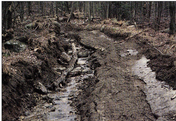
Figure 28. Forest Skid Trail Rutting Damage.
