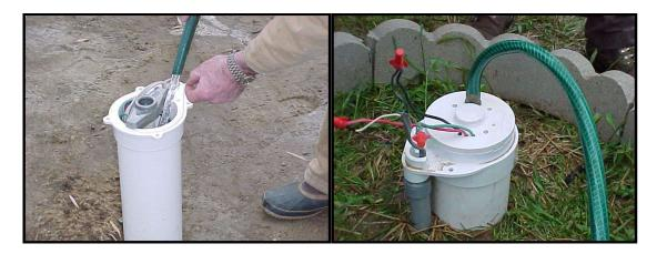
Some water well drilling contractors have extended the recirculation time to several hours. Extended recirculation has been shown to increase the effectiveness of the disinfection process. During extended recirculation a seal needs to be placed on the wellhead to keep contaminants from entering the well.
