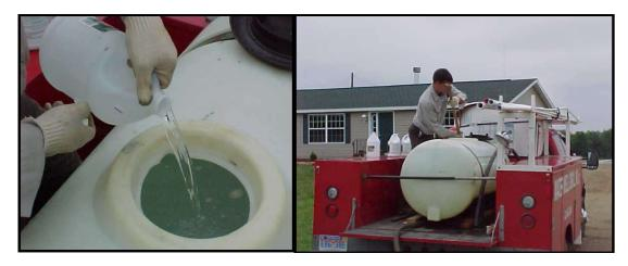
Use a well cleaning acid (carefully following manufacturers' instructions) to lower the pH of the chlorine solution being prepared in the bulk tank to 4 to 4.5. After the acid is added to the water in the bulk tank, the water must be agitated to assure uniform distribution of the acid. An air line, a recirculating pump, paddles, or other agitation methods should be used.
