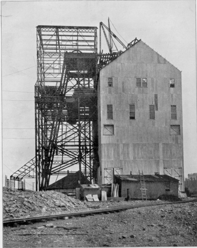
NO. 5 TAMARACK STEEL ROCK AND SHAFT HOUSE.
