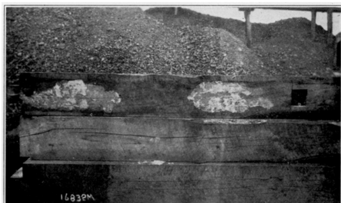
TIMBERS VERY MUCH WEAKENED BY DECAY DUE TO IMPROPER STORAGE. PROBABLY HALF THEIR VALUE GONE BEFORE THEY ARE PUT INTO SERVICE
