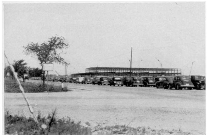
FIG. 1. Carnegie Steel Corporation Plant while under construction for the Chrysler Corporation on Mound Road
