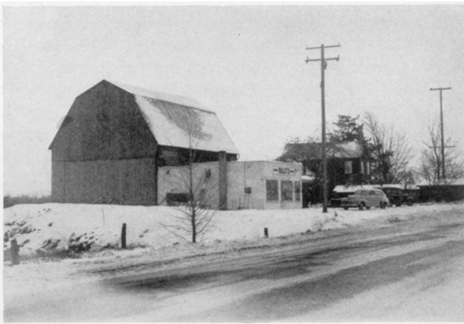
FIG. 1. An old farmstead barn converted into a store and shop dealing in building supplies
