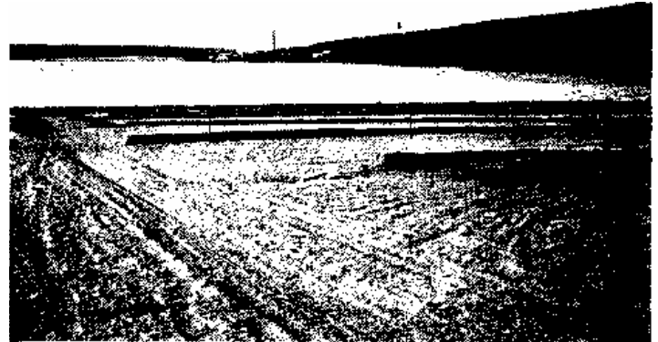
Figure 5. Strips of baled hay laid perpendicular to erosive winds. Distance between strips is one chain. View is southerly across Torch Lake. Note open expanse of water allowing uncontrolled movement of winds.
