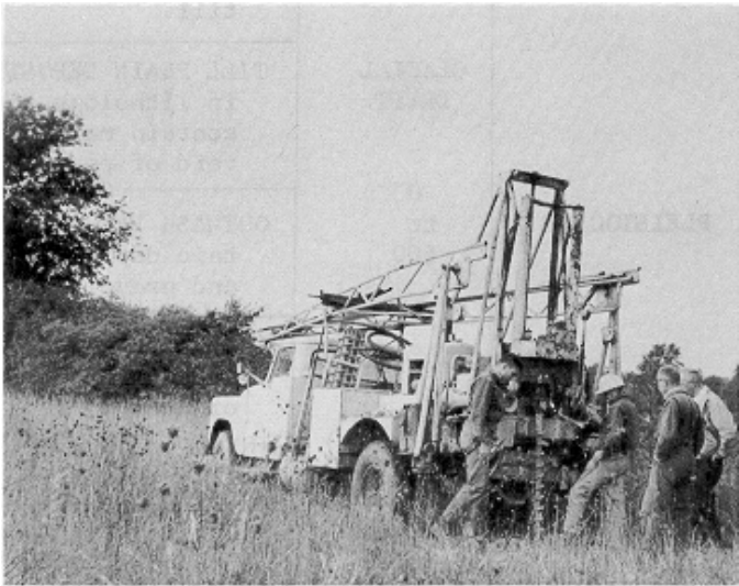
Drilling for geologic information.
