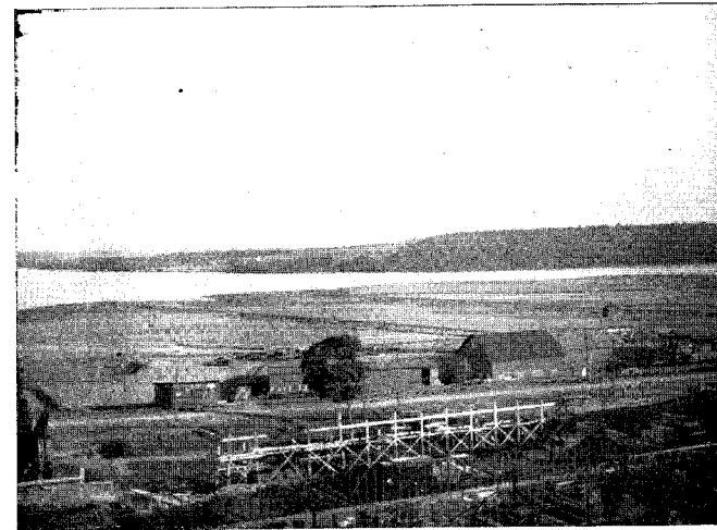
A. FOUNDATIONS OF THE TAMARACK RECRUSHING PLANT AND THE STAMP SAND IN TORCH LAKE.
